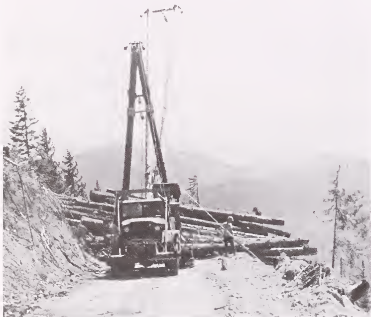
Figure 7.--Idaho jammer built on heavy truck chassis.
