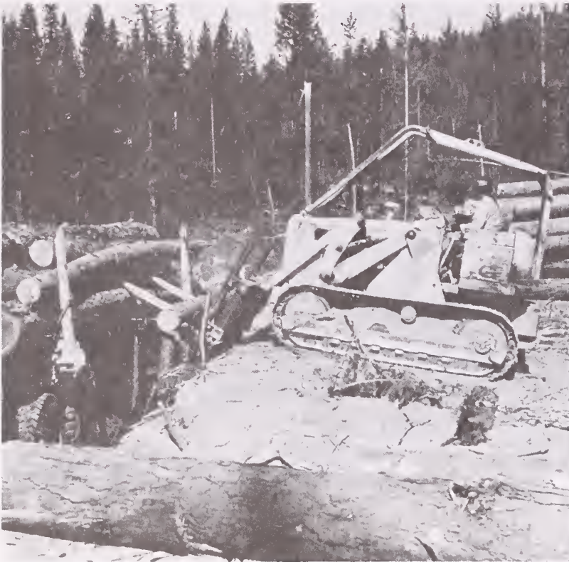
Figure 22.--Track-mounted front-end loader.
