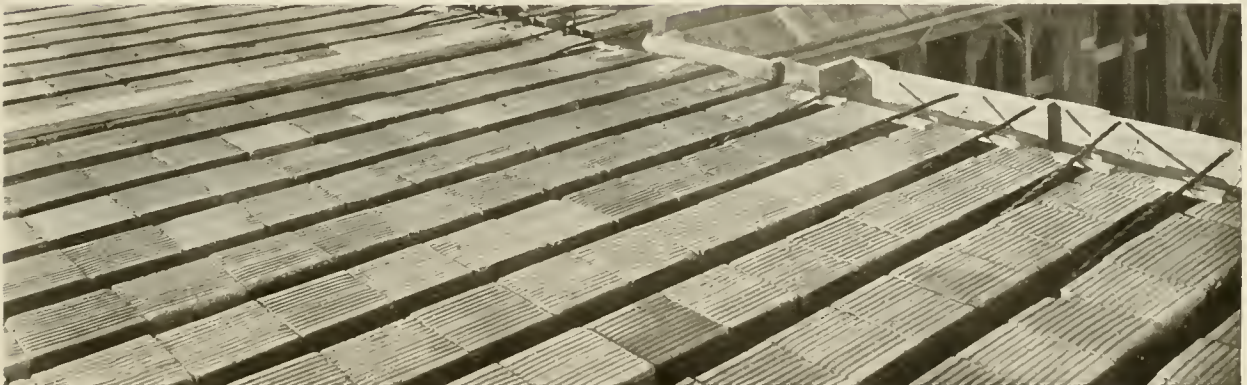
Hollow Tile floors are easy to lay. Illustration shows tile and reinforcing rods in place ready for the concrete, which forms joists and covering.
