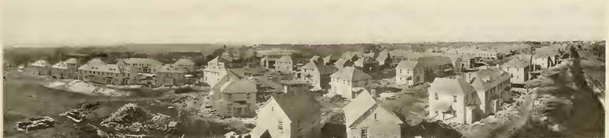
Hollow Tile houses erected by the United States Government Housing Corporation, New Brunswick, N. J. In the great emergency the United States Government found Hollow Tile the ideal available material, to solve the housing problem.
