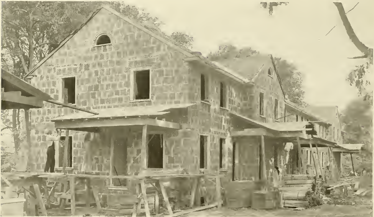
Hollow Tile house under construction, before stucco has been applied.
