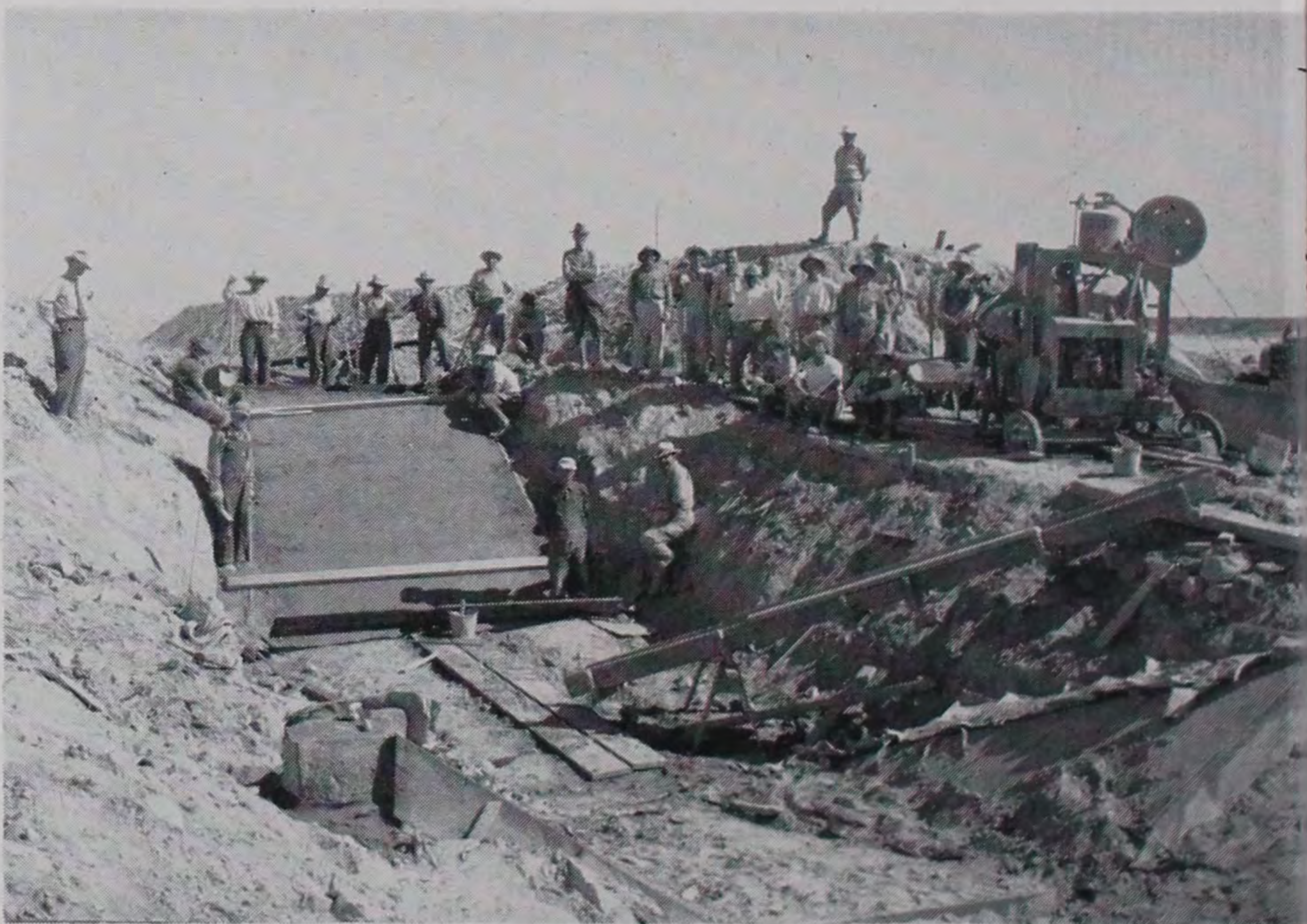
CONSTRUCTING A DROP
