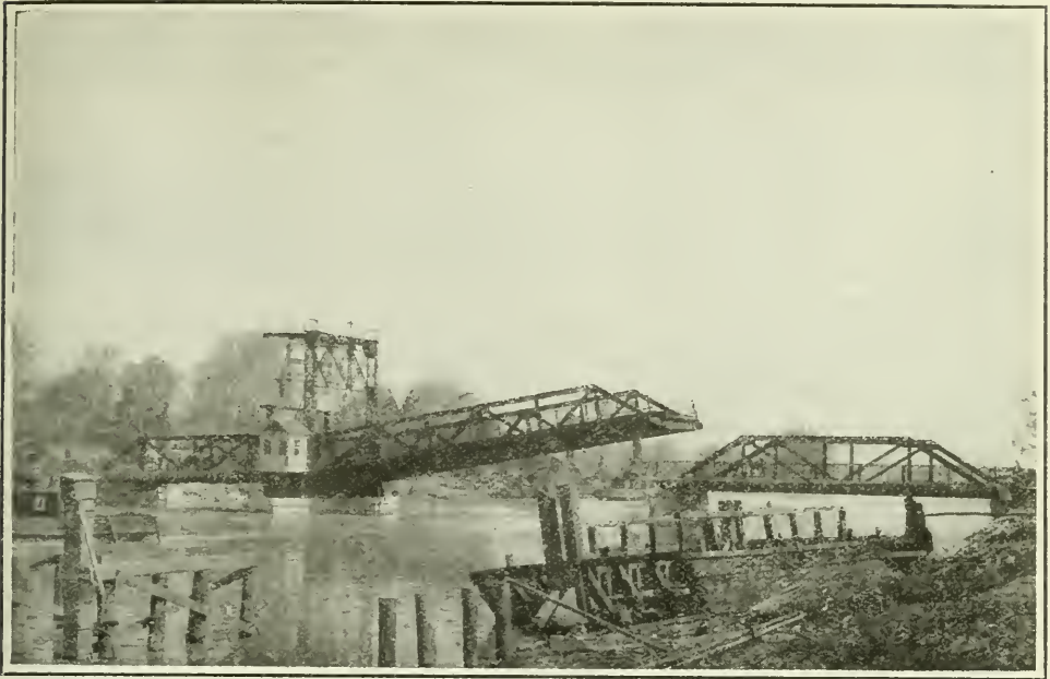
Chippawa Highway Bridge Closing, May 3, 1921
