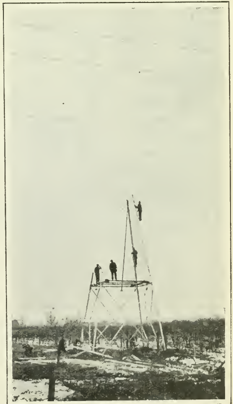
Combined Assembly and Erection of 1920-type Towers: Queenston-Burlington Line
