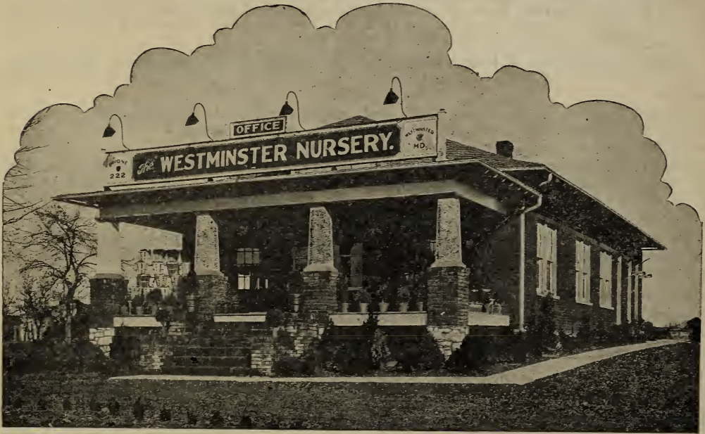
Our New General Offices and Sales Room with display gardens situated on Lincoln Highway to Baltimore, just outside of Westminister.
