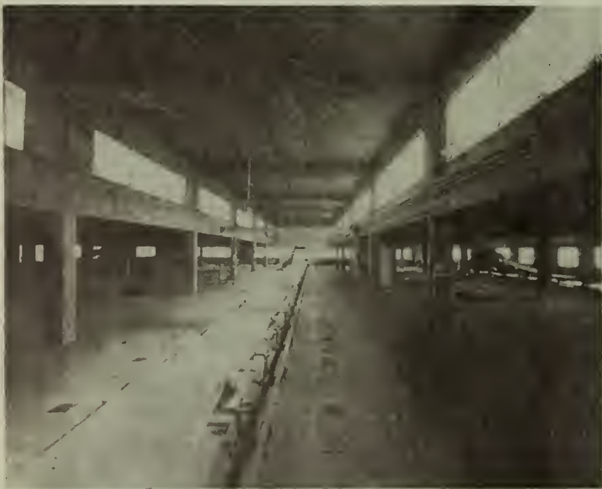
One of the belt conveyors in the new Murray Elevator at Kansas City, Mo., which is served by 2,000 feet of SUPER-SERVICE Rubber Belting.
