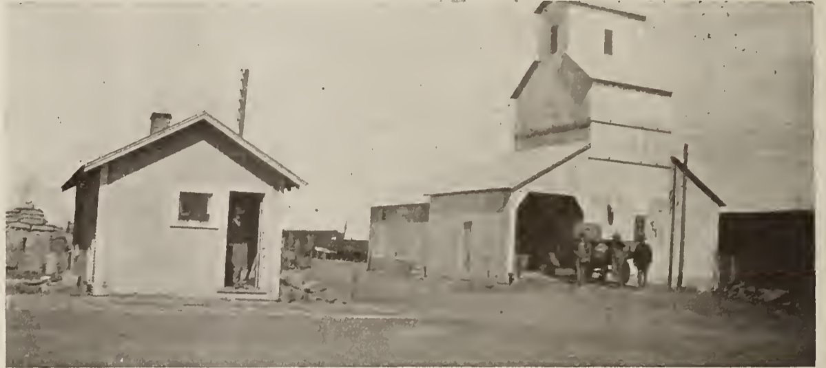
ELEVATOR AND WAREHOUSE PROPERTY OF THE SUDAN GRAIN & ELEVATOR COMPANY AT SUDAN, TEXAS
