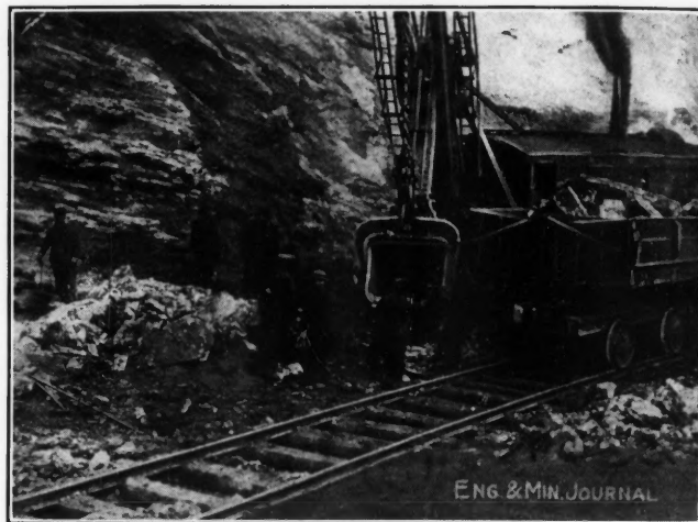
STEAM SHOVEL LOADING ROCK FROM THE BOTTOM OF THE GENOA PIT. THE DIPPER IS FILLED BY HAND
