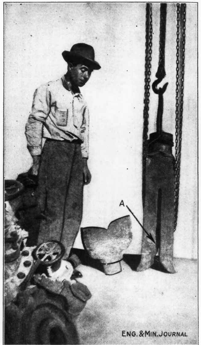
INSTRUMENT USED FOR EXTRACTING A REVERSED DRILL BIT
