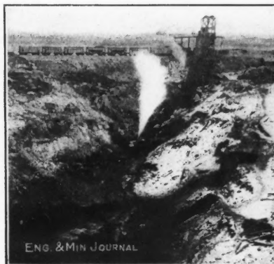
WHITE IRON LAKE MINE. A SMALL PROPERTY STRIPPED BUT MINED BY HAND WITH SKIP HOISTING
