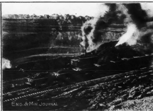
STRIPPING AROUND EDGE OF DEEP SUSQUEHANNA PIT, ON THE EDGE OF THE VILLAGE OF HIBBING
