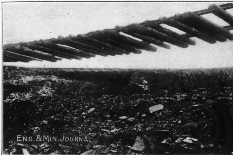
A RESULT OF THE SLICING SYSTEM, THE SURFACE CAVED FROM UNDER A RAILROAD TRACK
