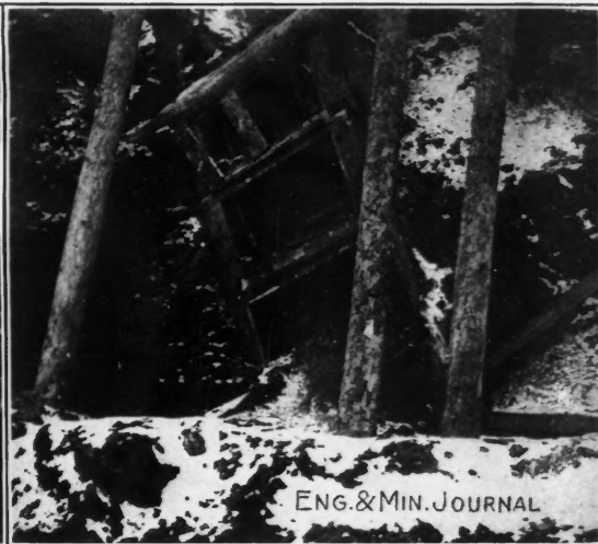
AN OLD INCLINED SHAFT IN THE GENOA PIT UNCOVERED BY THE STEAM SHOVEL
