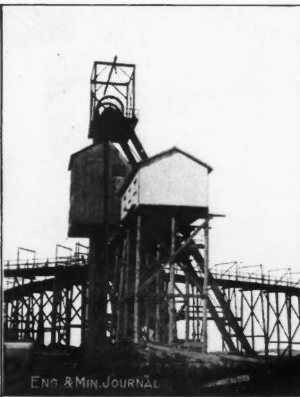
MODERN STEEL TWO-POST HEADFRAME AT MORTON MINE. NOTE FOUR DIFFERENT TRESTLES
