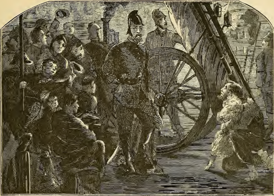
THE FIRE ESCAPE.
