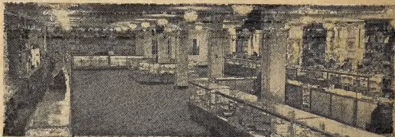
INTERIOR OF NEW POST EXCHANGE WING
