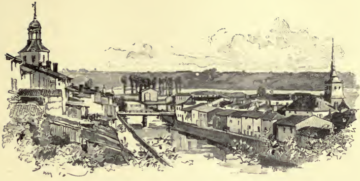
BRIDGE OVER THE AIRE AT VARENNES.
