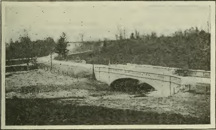
In Wisconsin the Federal Money is Going Into Such Works As This Road and Bridge.
