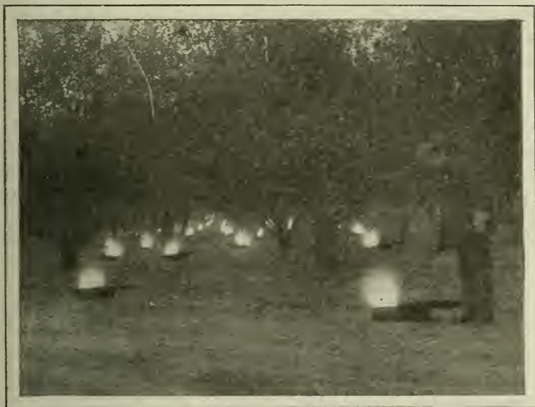
A Popular Type of Oil Orchard Heater in Operation.
