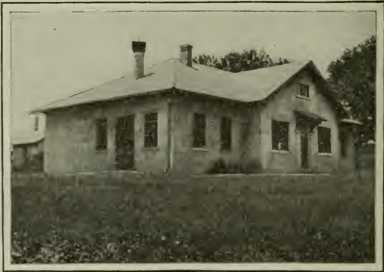
FIG. 4.—The Milk House is of Sanitary Construction.
