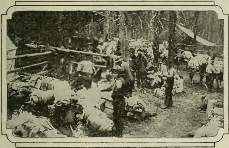
Backing Up the Fire Fighters.
