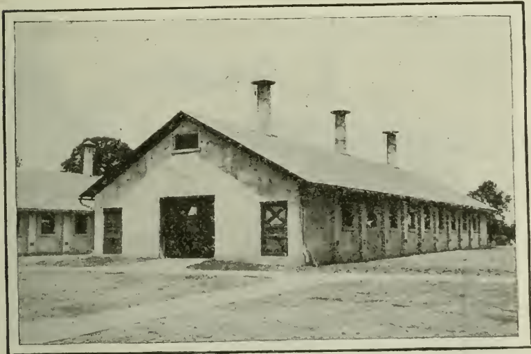
FIG. 2.—Cows are Housed in Hollow-Tile Stables, with Concrete Floors and Plenty of Light and Air.
