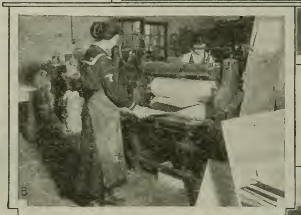
B. Gluing Up Plywood.
