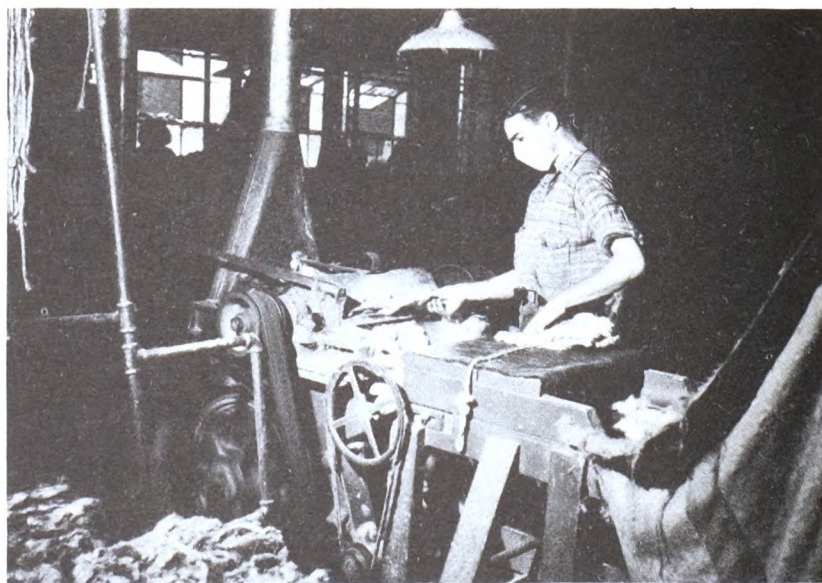
PH 3013. The effectiveness of the exhaust ventilation system at this fur cutting operation is shown by the dust-laden lighting fixtures.
