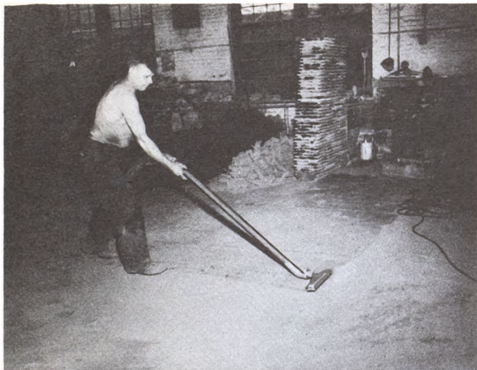
PH 3020-C. This unusually well-lighted and well-ventilated foundry has a concrete floor which is vacuum-cleaned each day, taking up every bit of sand and dust.
