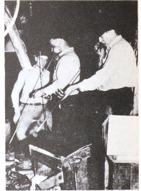
PH 829-M5. A team making glass bottles in a glass factory. The heat is intense, so the workers are supplied with cooled air.
