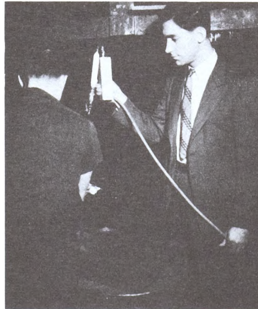
PH 2964. Industrial Hygiene engineer taking air samples where exposure to poisonous fumes is suspected.
