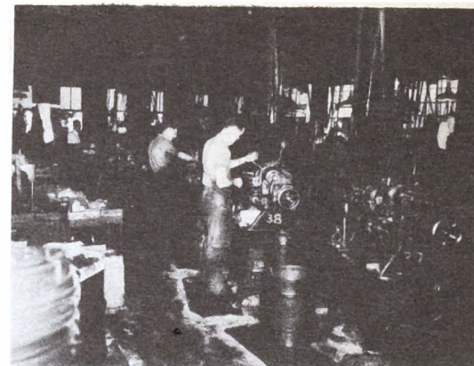
PH 2975-D. Poor lighting and overcrowding of machines increase the hazards of industrial work.
