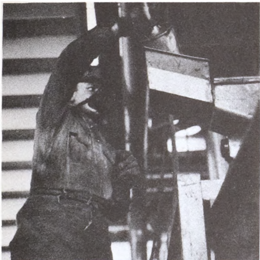
PH 3055-E. On jobs where exhaust ventilation is impossible, workers must wear approved masks to prevent exposure to dangerous materials.
