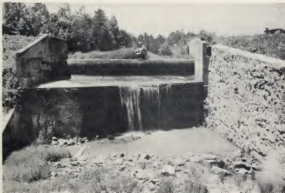
Figure 3.--Spillway of Franklinton Dam.
