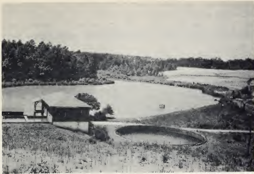
Figure 2.--General view of Franklinton Dam and Reservoir.
