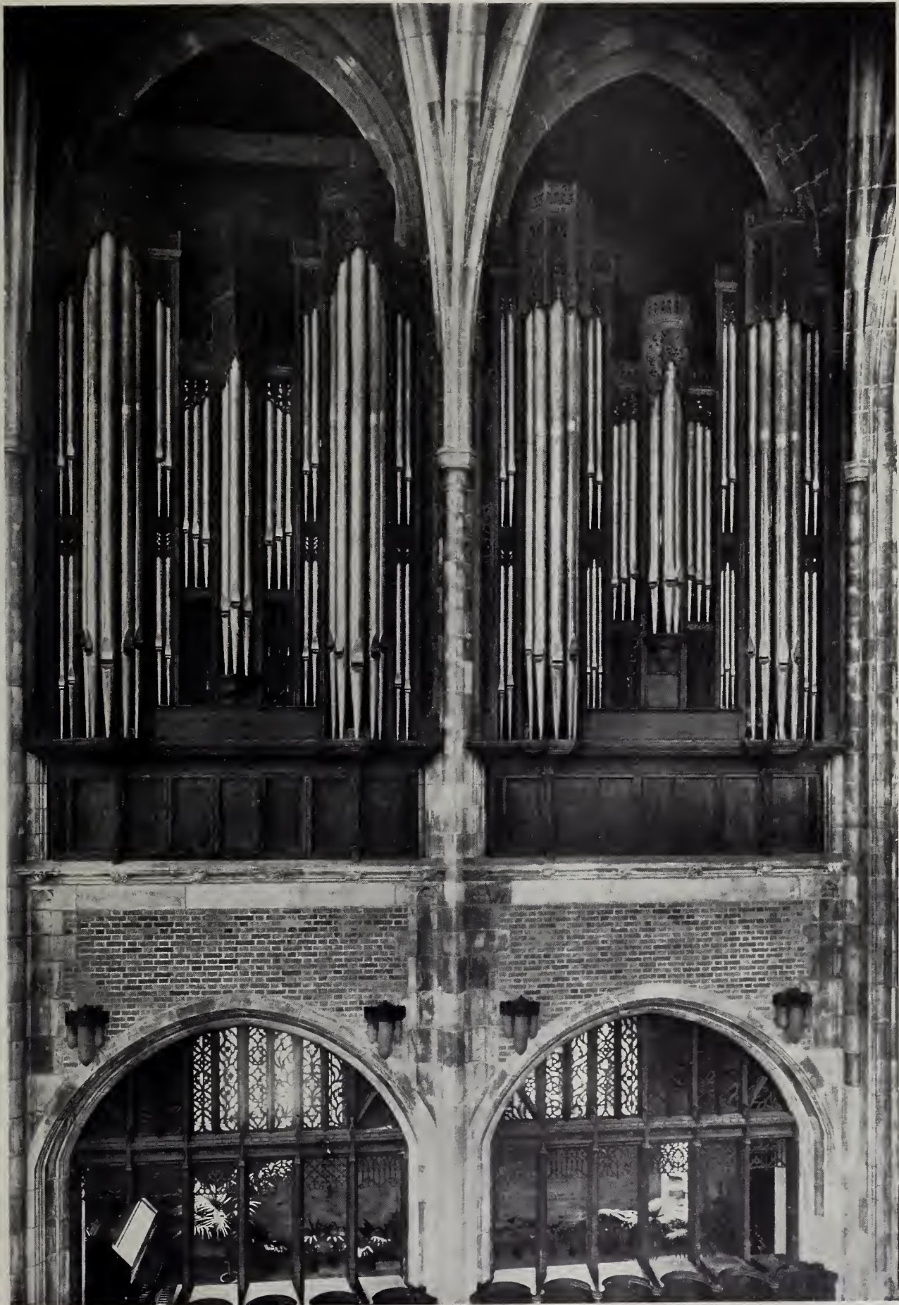
ORGAN CASES, CHAPEL OF THE U. S. MILITARY ACADEMY, WEST POINT, N. Y. CRAM, GOODHUE & FERGUSON (NEW YORK OFFICE), ARCHITECTS
