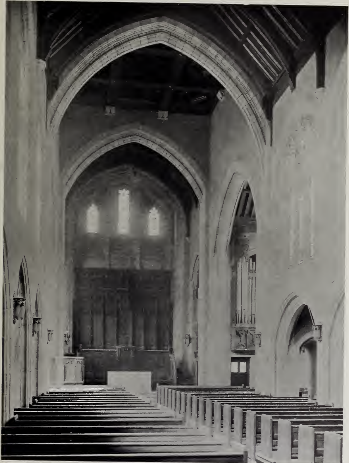
SAGE MEMORIAL CHURCH, FAR ROCKAWAY, NEW YORK CRAM, GOODHUE & FERGUSON (NEW YORK OFFICE), ARCHITECTS
