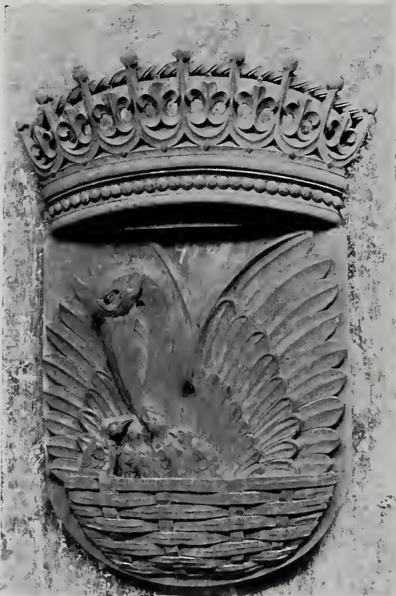
PELICAN IN PIETY FROM CRESTING, CHAPEL OF THE INTERCESSION
