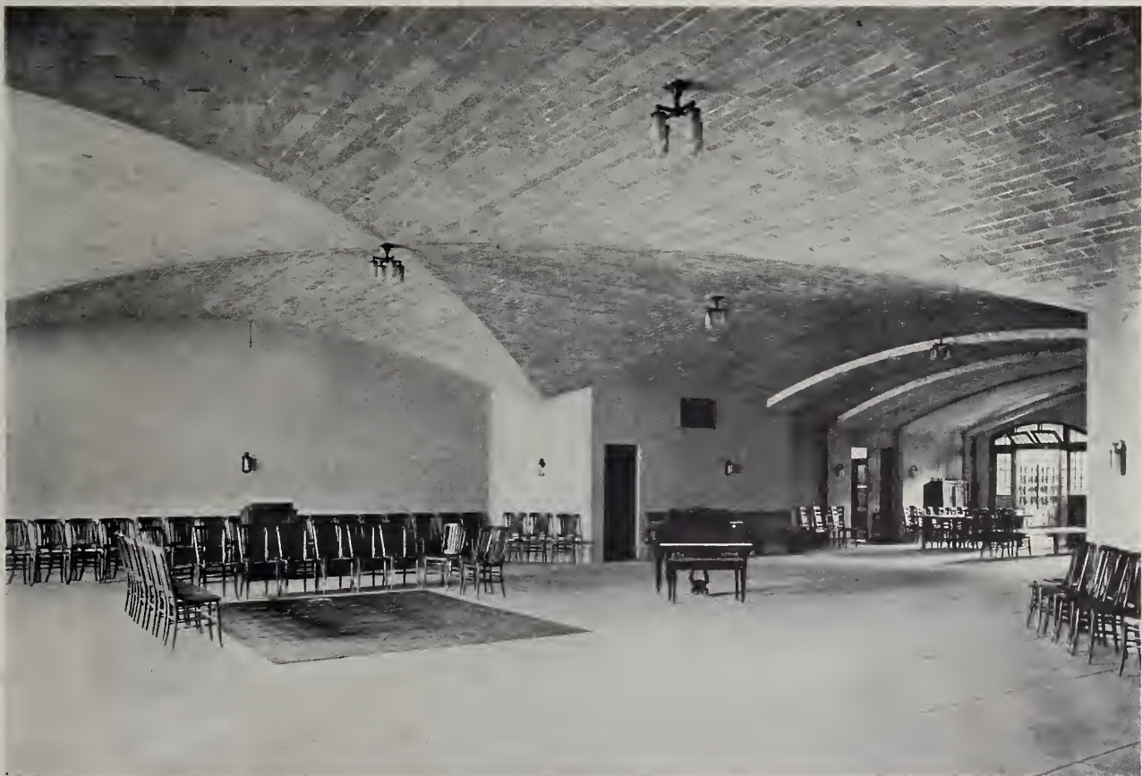
ASSEMBLY ROOM IN BASEMENT
