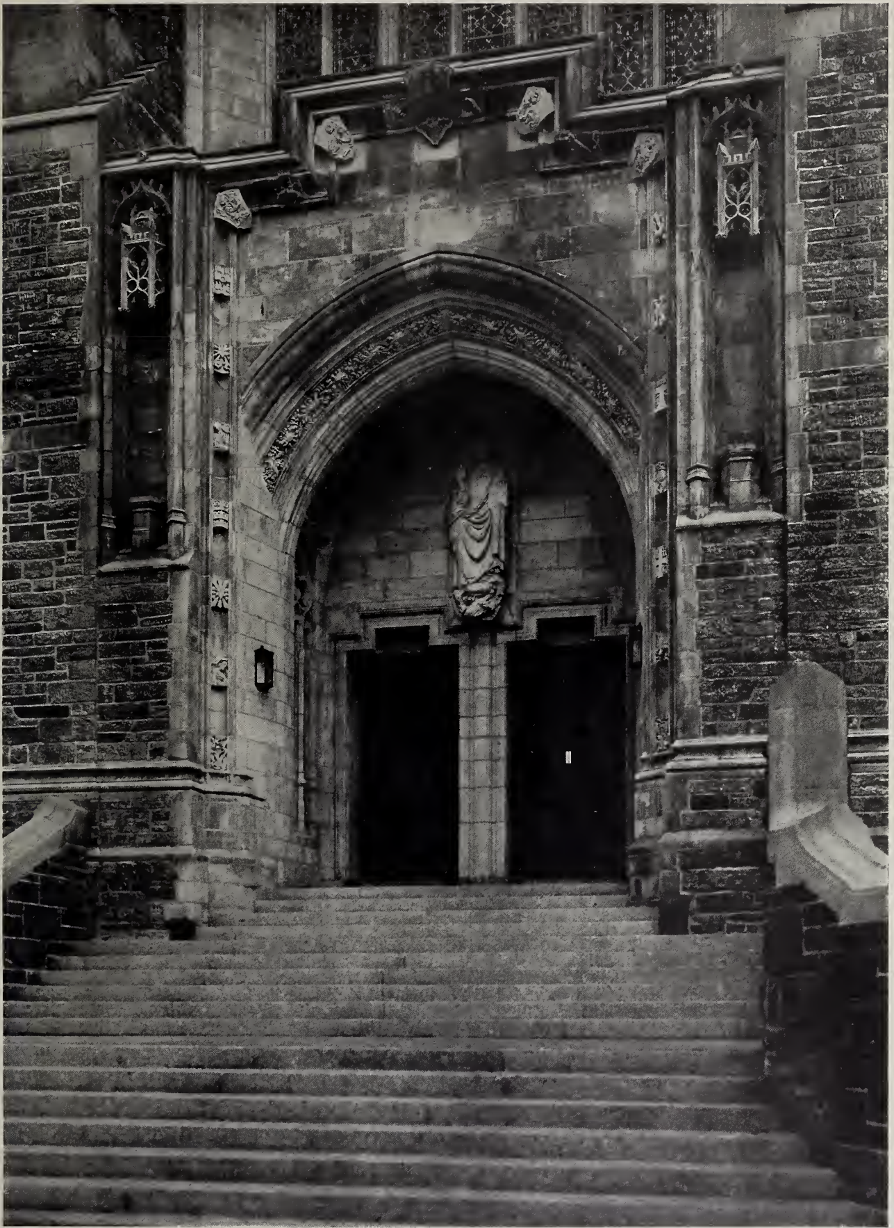
CHAPEL OF THE INTERCESSION, NEW YORK BERTRAM GROSVENOR GOODHUE; CRAM, GOODHUE & FERGUSON (NEW YORK OFFICE), ARCHITECTS
