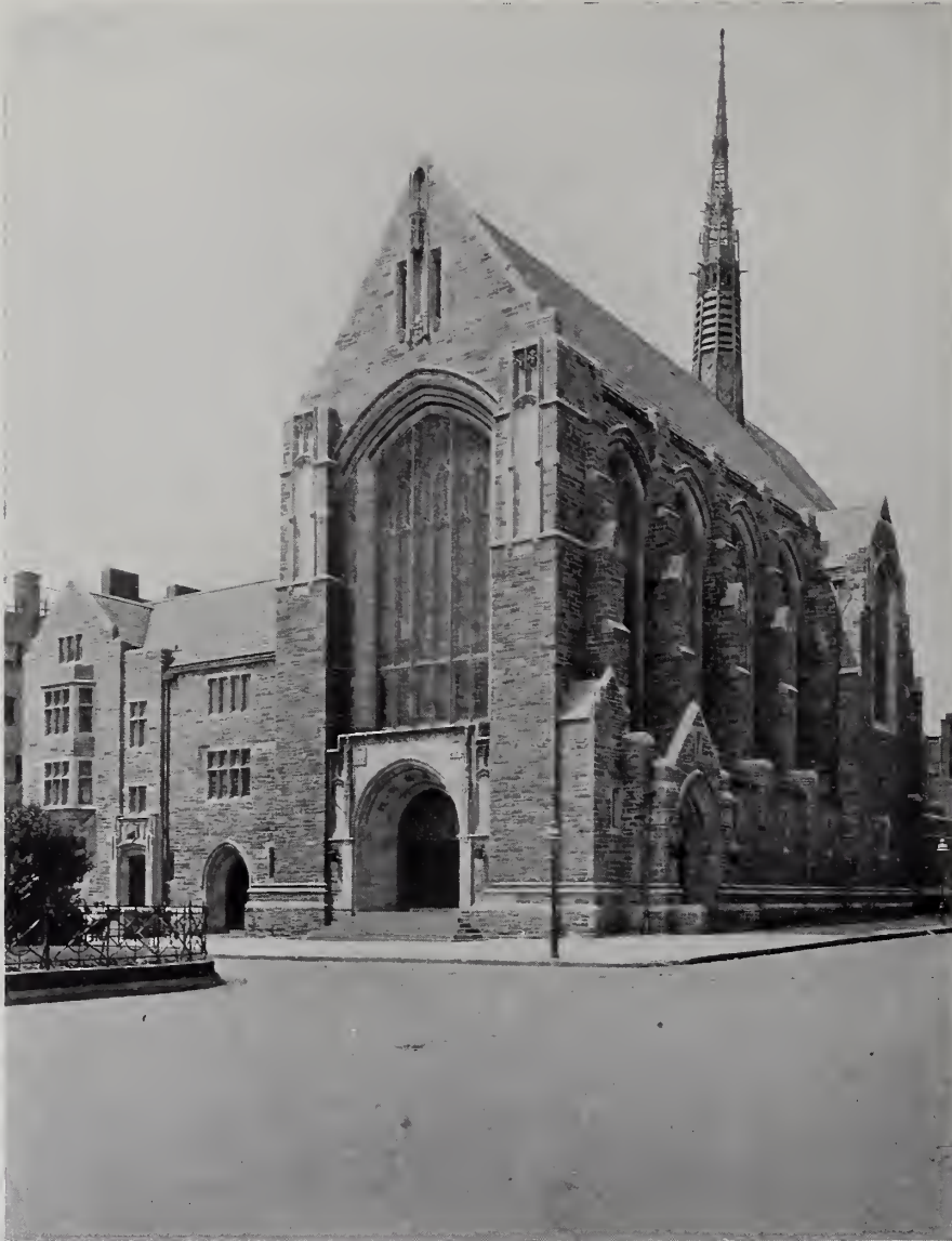
SOUTH CHURCH (DUTCH REFORMED), NEW YORK The Flèche is of cast lead.
