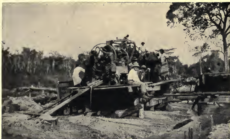
WASHING OUT GRAVEL
