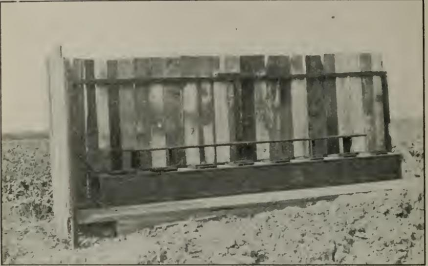
Flyproof toilet in course of construction according to plans furnished by the Commission. The lids over holes are on hinges and are forced to fall by plank in back.
