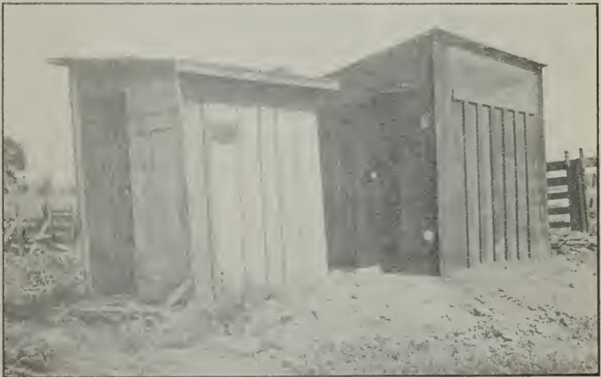
An old, non-flyproof toilet to the left, and a new, screened, flyproof toilet with automatically closing door to the right: the latter built according to plans furnished by Commission.
