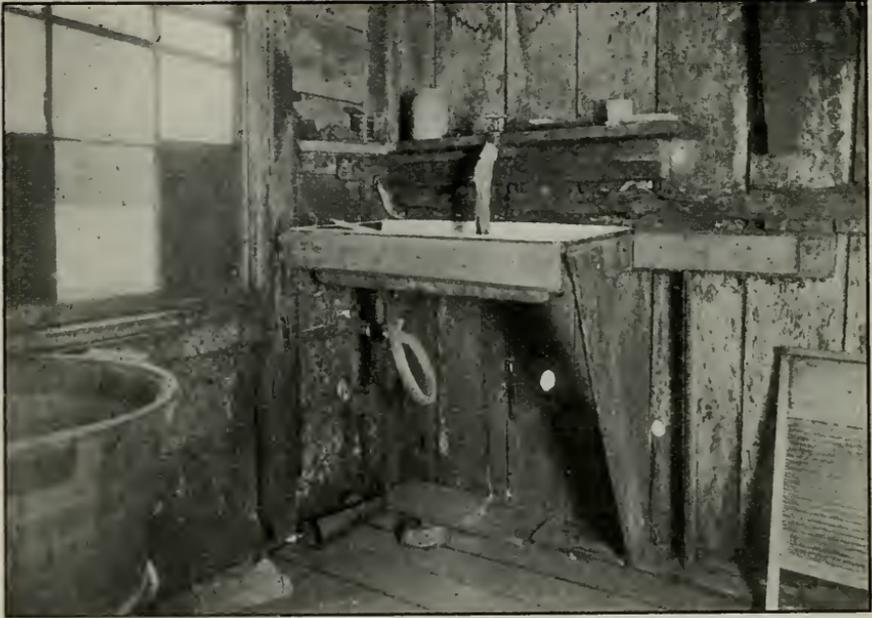
A piece of leaky rubber hose used as substitute for broken pipe. The faucet is badly in need of repair.
