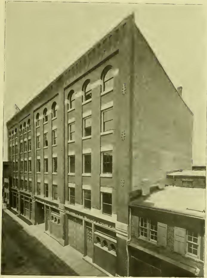
STOCK, SHIPPING AND SALESROOM BUILDING
