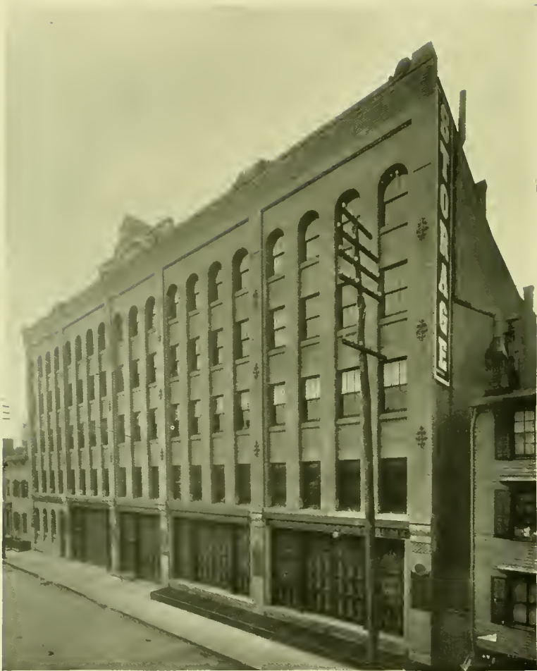
NEW STORAGE WAREHOUSE
