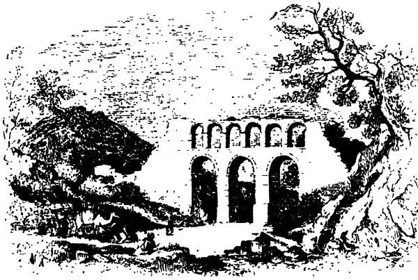
AQUEDUCT AT EPHESUS.
