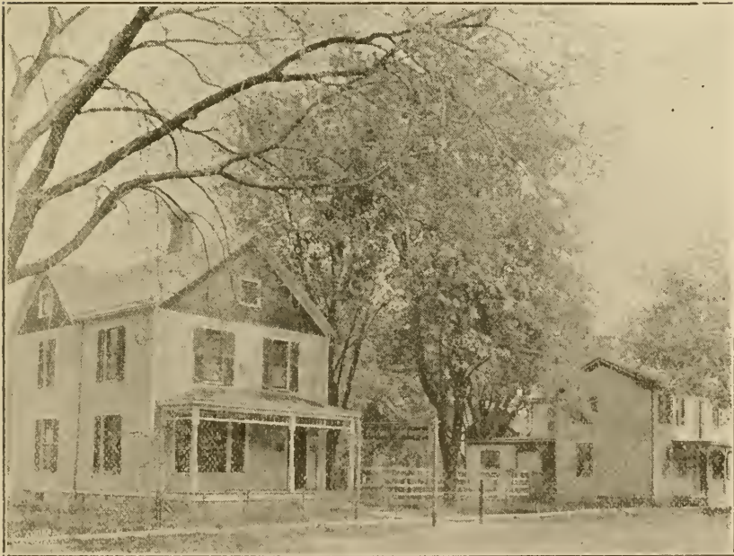
OFFICE AND HOSPITAL.
