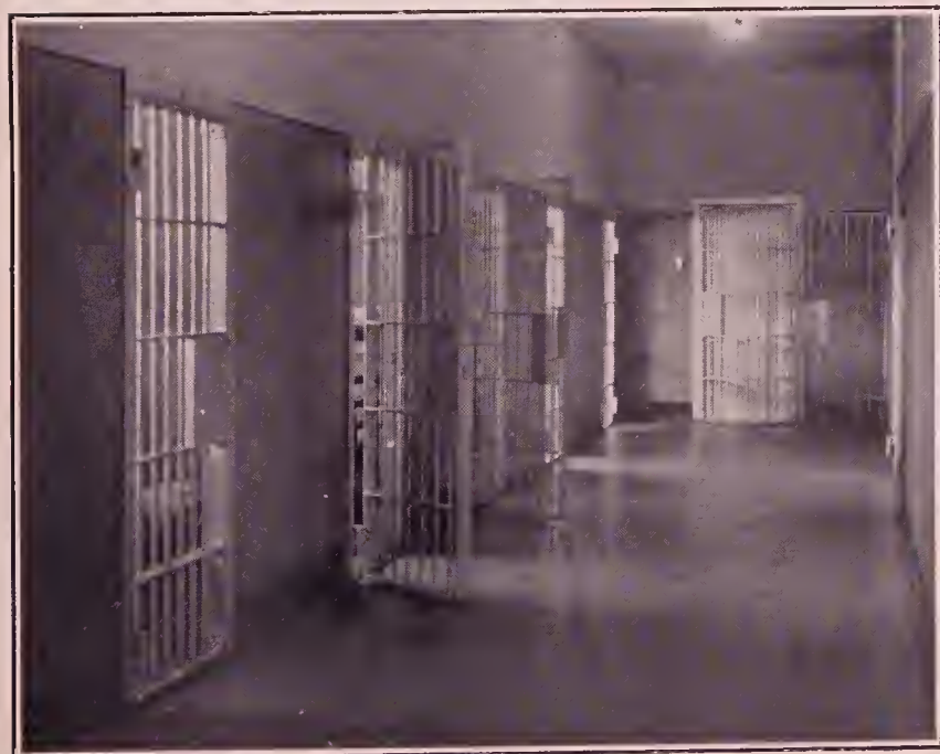
NORTH CORRIDOR, CITY JAIL
