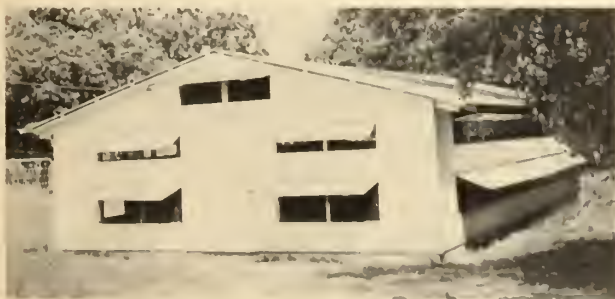
FIGURE 33.—Shutters hinged to serve as shades.
