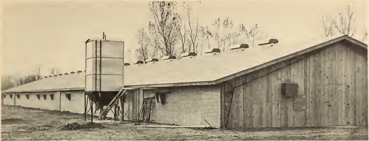
FIGURE 13.—Insulated windowless A-frame laying house with fans on the sidewall, prefabricated ridge vents, and bulk-feed storage bin. In foreground at gable end is egg-cooling machine and door for removing cased eggs from egg-cooling room.
