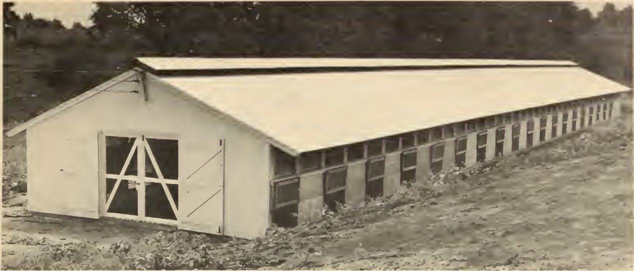
FIGURE 16.—A 24- by 160-foot laying house with reflective roofing, continuous ridge ventilators, floor-level windows, and large end doors.
