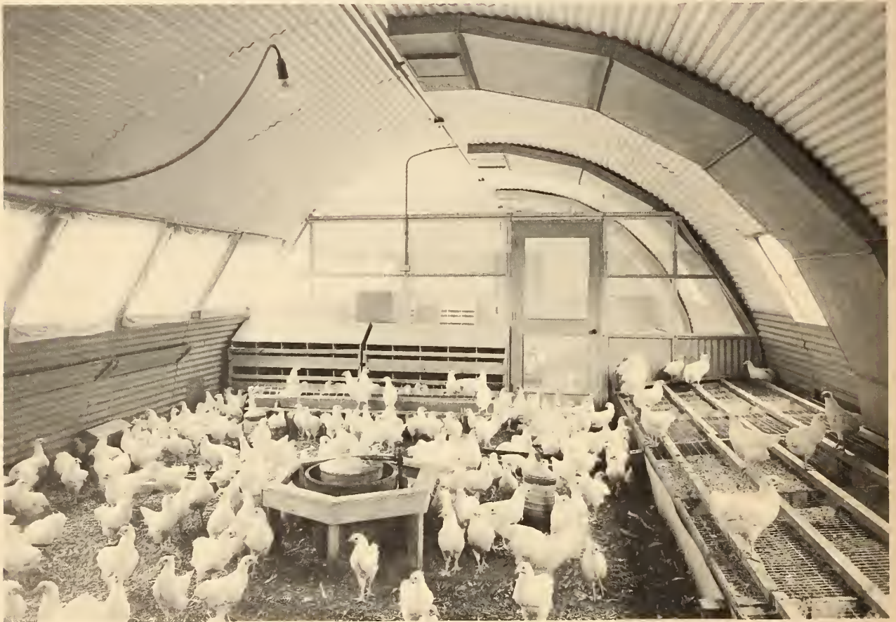
FIGURE 37.—Droppings pit built along rear wall in a prefabricated metal laying house.
