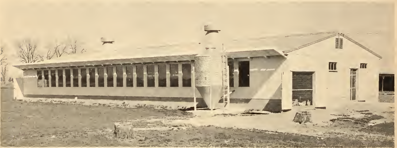
FIGURE 12.—Solar laying house showing large insulating glass windows with sunshade designed to shade windows in summer but not in winter.
