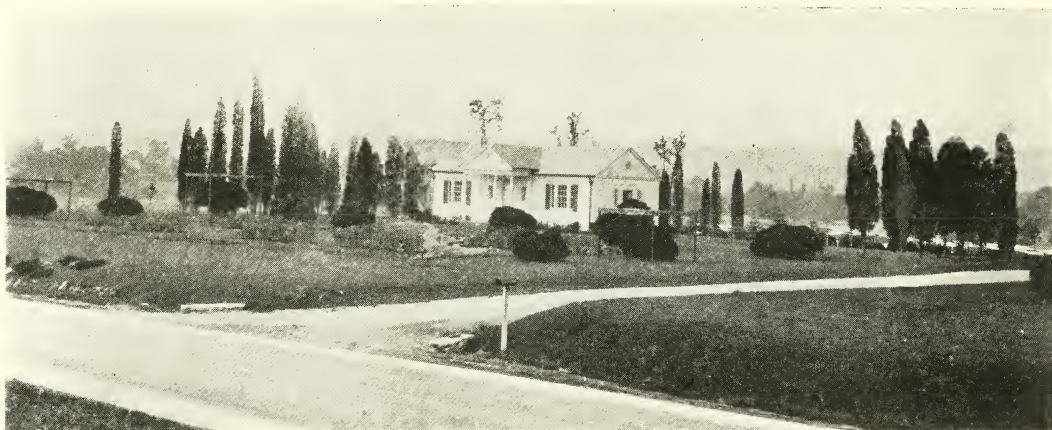
Main entrance, and front of area south of avenue dividing plantation, showing some larger Boxwood and office building, with Boxwood also in the background.
