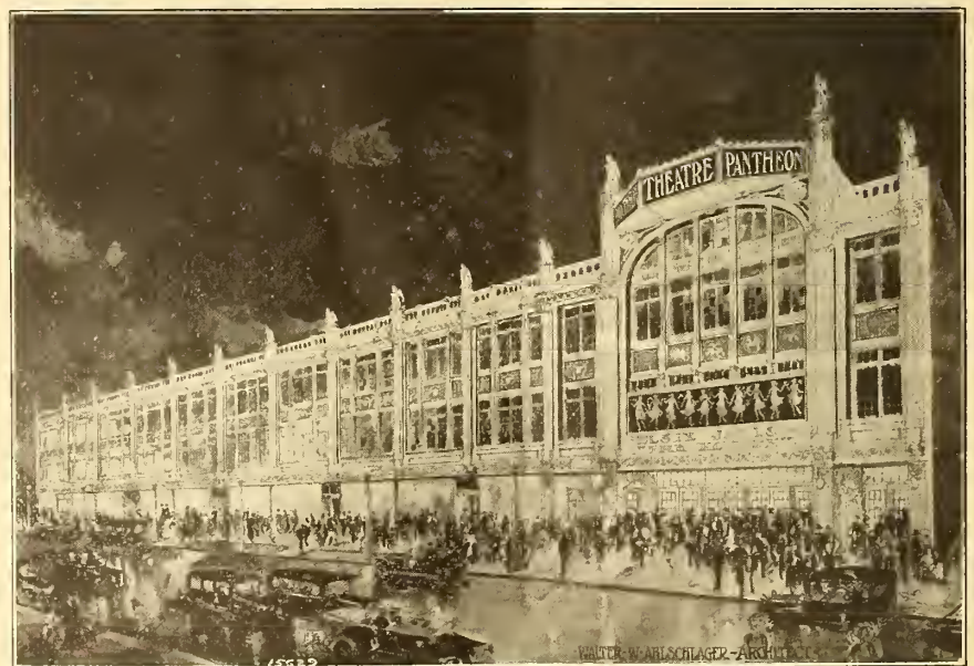
Pantheon Theatre, new $550,000 house being erected at Sheridan Road and Wilson avenue, Chicago, by Lubliner and Trinz. The theatre will open in the fall.
