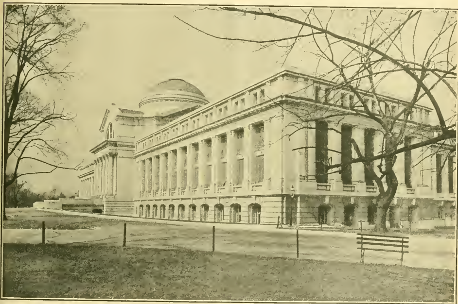
FIG. 1.—United States National Museum, Natural History Building, viewed from S.E., showing the South front, the outer end of the East wing, and the beginning of the East range.
