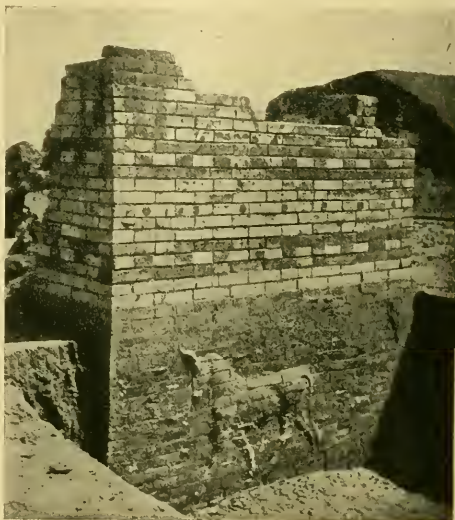
FIG. 1.—Enamelled wall length of the Ishtar Gate. From "The Excavations at Babylon."
