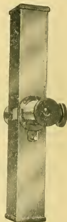
FIG. 6.—Alder and Cochrane's extinction pyrometer.
