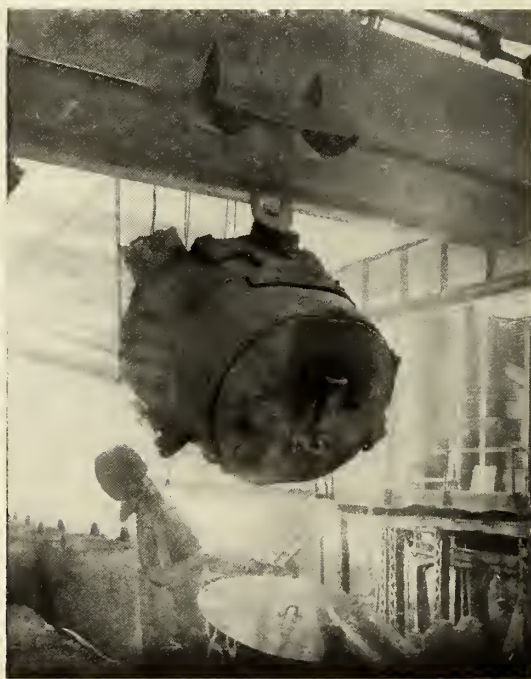
THE HUGE LADLE DANGLING FROM THE CRANE BY A SINGLE HOOK.
