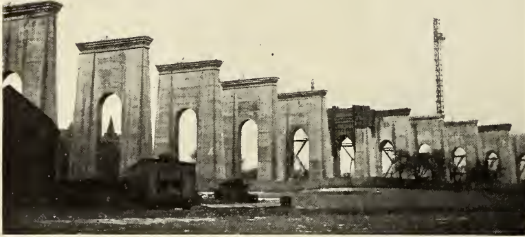
THE CONCRETE LEGS OF THE VIADUCT LEADING TO THE GREAT ARCH.
