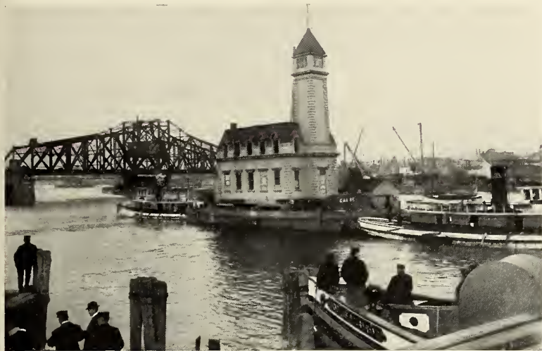
THE FIRE-BOAT HOUSE SHIPPED UPON A SCOW AND TOWED TO A NEW SITE A MILE UP-STREAM.
