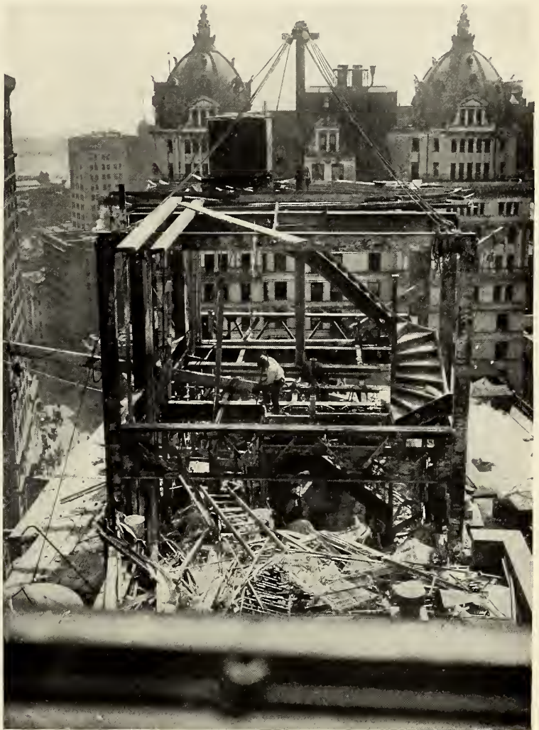
REDUCING A 300-FOOT OFFICE-BUILDING TO JUNK.
