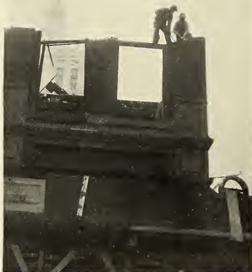
PRYING OFF BRICKS WITH THE PINCH-BAR.
