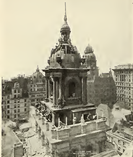
RIPPING OPEN THE TOWER OF THE SKY-SCRAPER.
