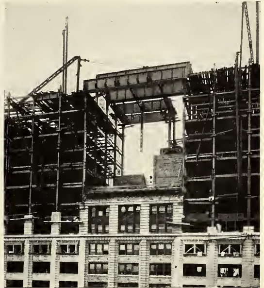
THE BRIDGE OVER THE OLD BUILDING. THE FIRST HANGER IN PLACE.
