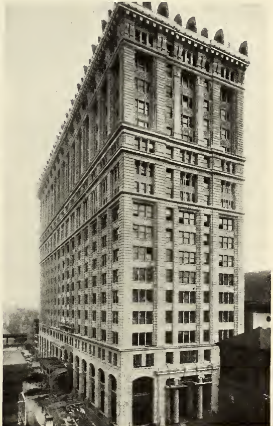
"IMPOSSIBLE TO TELL WHERE THE OLD BUILDING STOPPED AND THE NEW BEGAN."
