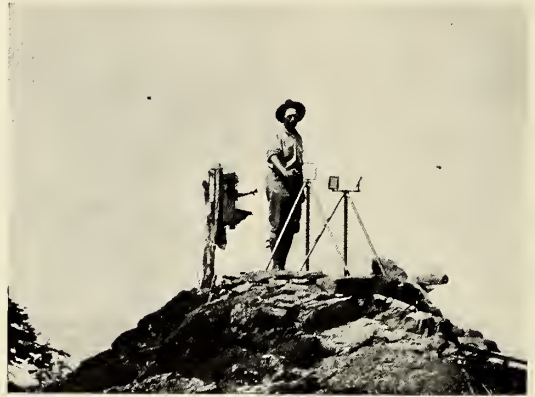
A FOREST RANGER USING A HELIOGRAPH TO SIGNAL TO OTHER LOOKOUT STATIONS.
