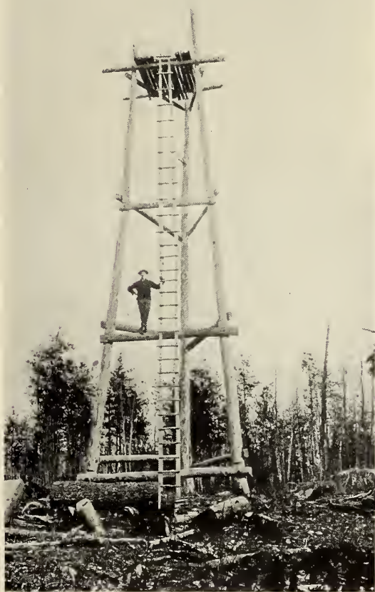
A WATCH-TOWER BUILT OF LOGS.
