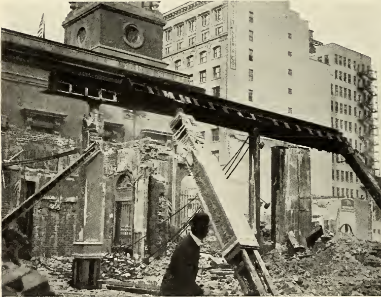
PULLING DOWN THE STEELWORK WITH ROPE AND TACKLE.
