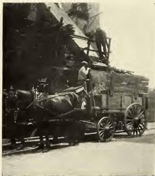
LOADING A CART AT THE BRICK CHUTE.
