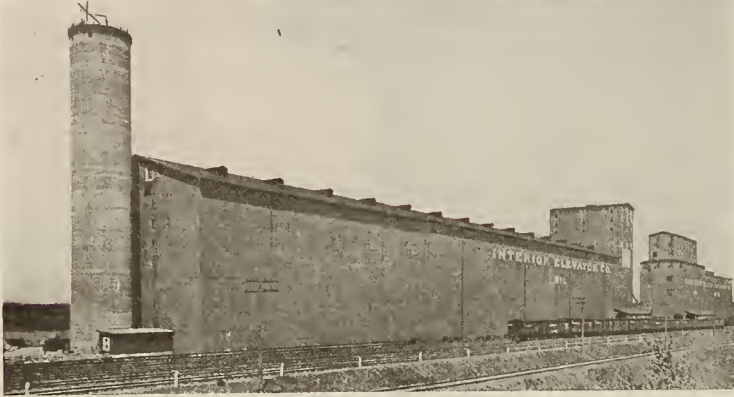
THE FIRST CONCRETE GRAIN TANK IN AMERICA Experimental tank erected at Minneapolis in 1899 for the purposes of study and experiment
