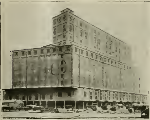
Manchester Ship Canal Elevator Manchester, England Capacity 1,500,000 Bushels Completed 1914
