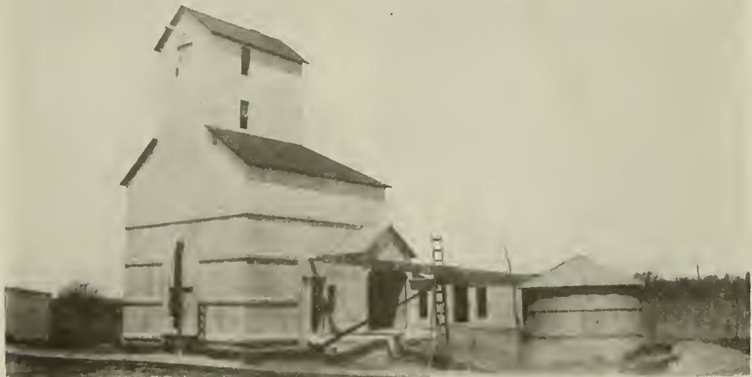
ELEVATOR OF THE J. D. COLLINS GRAIN COMPANY PLYMOUTH, KAN.
