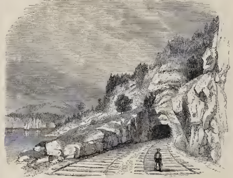
TUNNEL AT ANTHONY'S NOSE.
