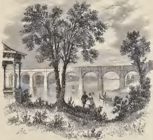
THE HIGH BRIDGE.*
