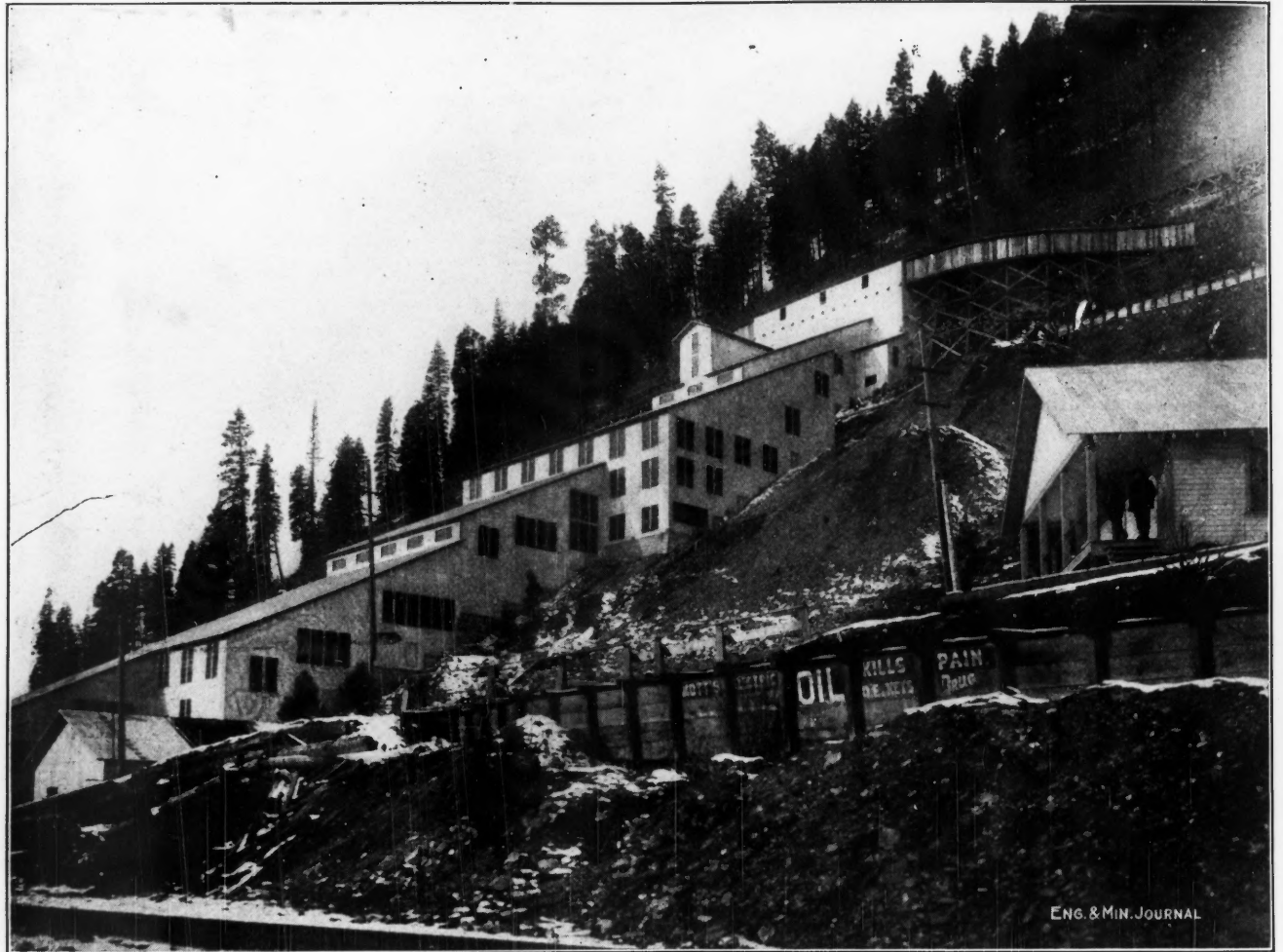
NEW 500-TON COPPER CONCENTRATOR OF THE NATIONAL COPPER CO., NEAR MULLAN, IDAHO Copper minerals are recovered by concentration and flotation, a high extraction being made.
