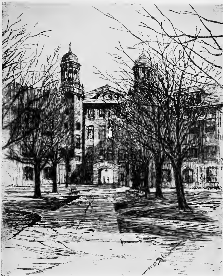
THE ENGINEERING QUADRANGLE
