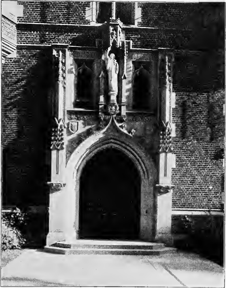
THE DOORWAY OF THE MARTHA COOK BUILDING
