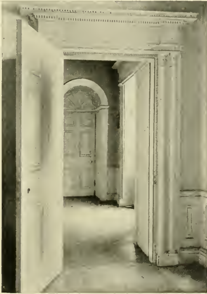
DOORWAY IN MANIGAULT HOUSE
