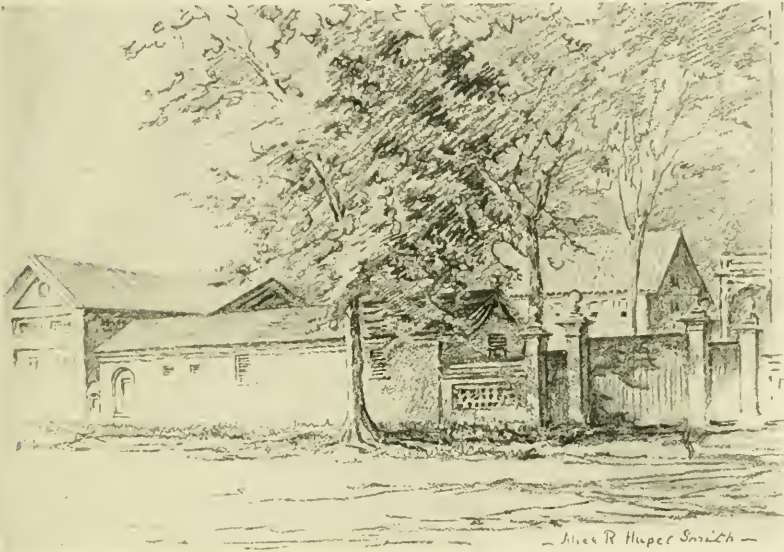
CARRIAGE-GATE AND OUTHOUSES OF JEFFERSON BENNETT RESIDENCE
