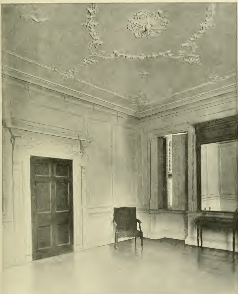
DETAIL OF ROOM IN MILES BREWTON'S HOUSE, FIRST FLOOR
