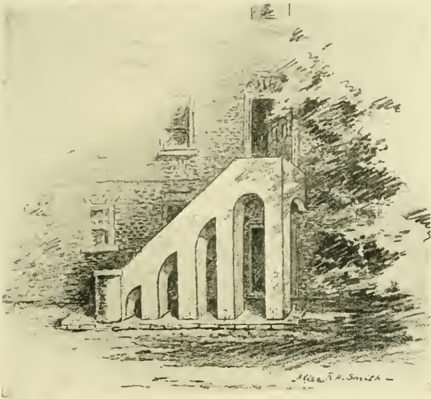
BACK STEPS OF ST. PHILIP'S PARSONAGE, BUILT ABOUT 1770
