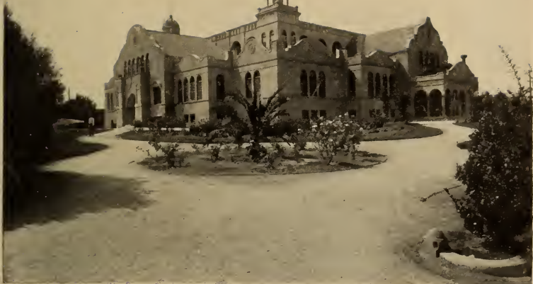
HIGH SCHOOL, RIVERSIDE, CALIF. In modern Mission architecture.
