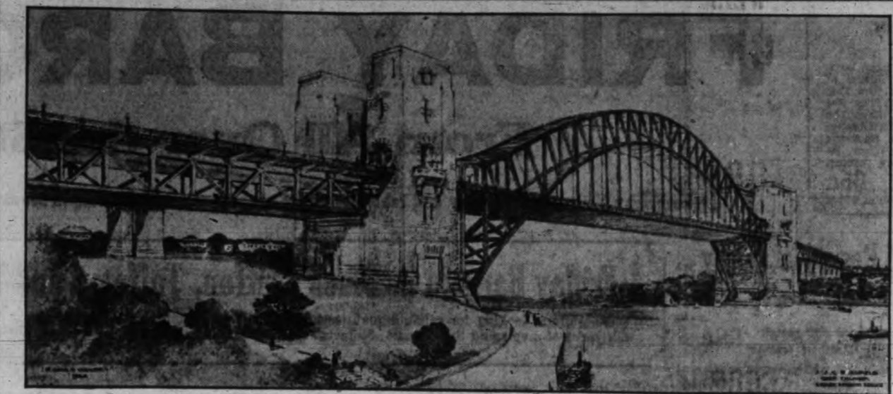
Details of the largest bridge in the world, which is to be built across the harbor of Sydney, Australia, by Dorman Long & Company, England, were given by G. C. Imbault, consulting engineer who prepared the design. Mr. Imbault passed through Victoria last week on R.M.S. Niagara. The bridge will cost $21,000,000 and will be 6,588 tons in weight when completed. It will span Sydney harbor from Dawes Point to the North Shore and in length will be 2,000 feet with a width of 160 feet. It will be specially constructed for use of railway, street car, vehicular and pedestrian traffic.
