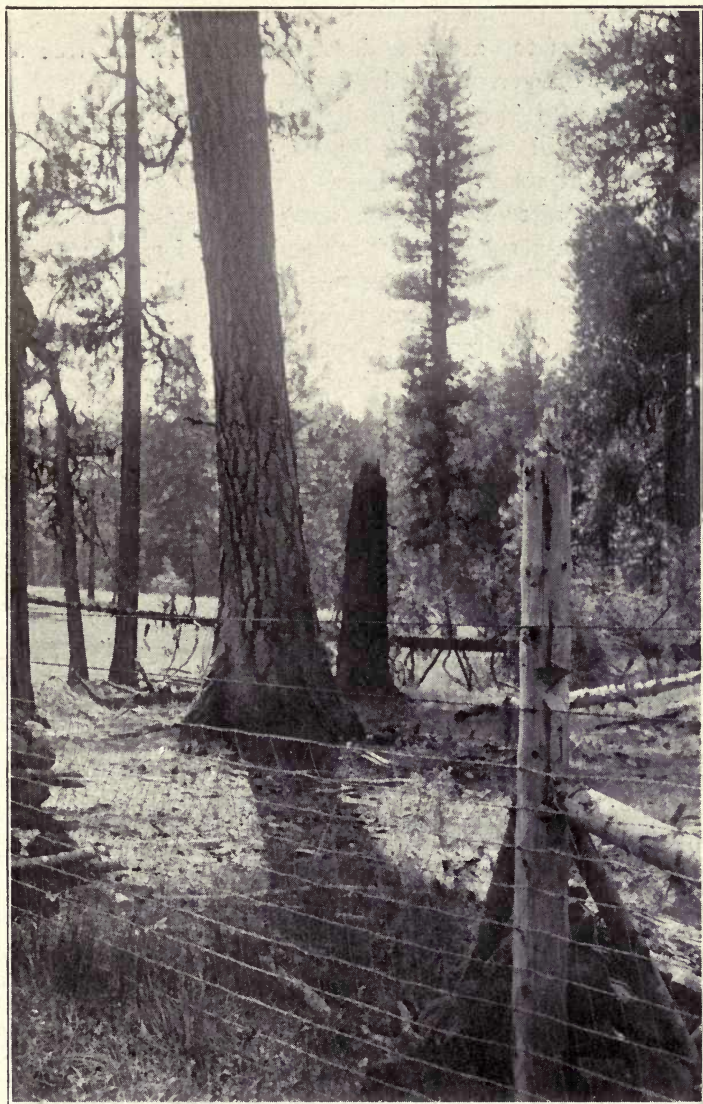
Built by the Forest Service in Oregon.
