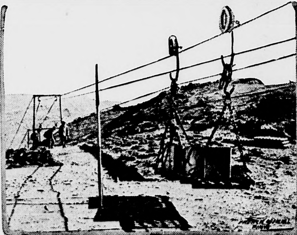
This French official photograph shows the Col de Cegel in Macedonia, where ammunition is transported up the mountain side by means of carriages suspended from an aerial trolley.
