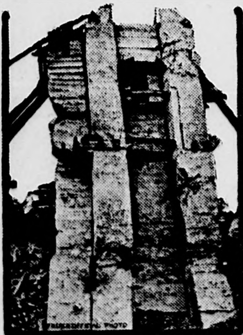
This picture of a German concrete observation post at a point in France now in the hands of the French gives an idea of the elaborate manner in which the Germans make war.
