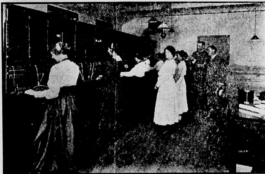
THE NEW CAMP DEVENS SWITCHBOARD
