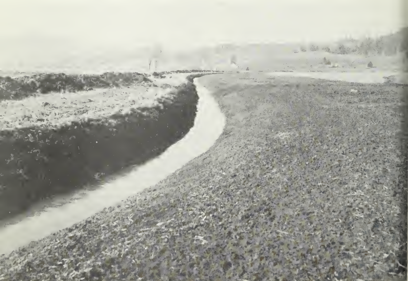
Open drain - One slope flattened with spoil spread. (Photo No. 0-702-3)
