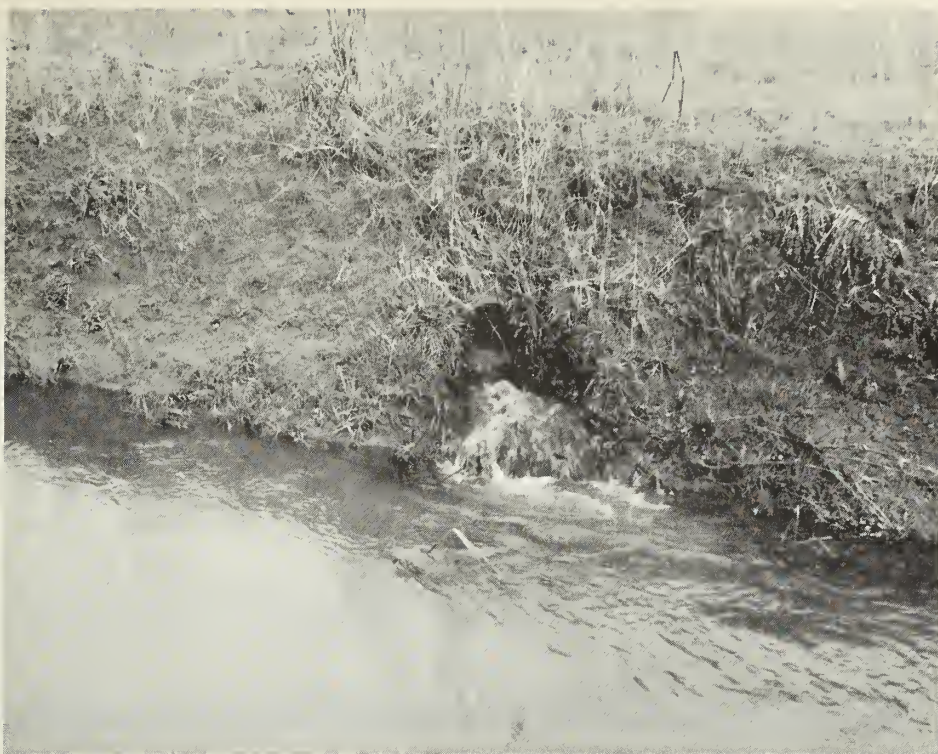
Benton County - Tile drain outletting into a natural drainage channel. Note height of outlet above water surface. (Photo No. 0-798-12)
