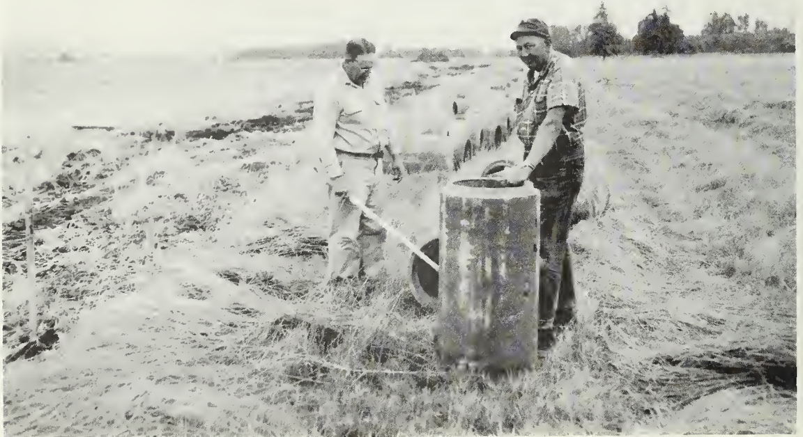
Linn County - Fifteen-inch concrete pipe, tongue and groove ASTM C-118 type. Used in deeper trenches or for larger subsurface main lines. (Photo No. 0-1295-6)
