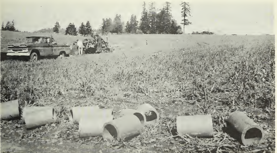
Clackamas County - Six-inch clay tile, standard grade, used in main line. (Photo No. 0-1576-9)
