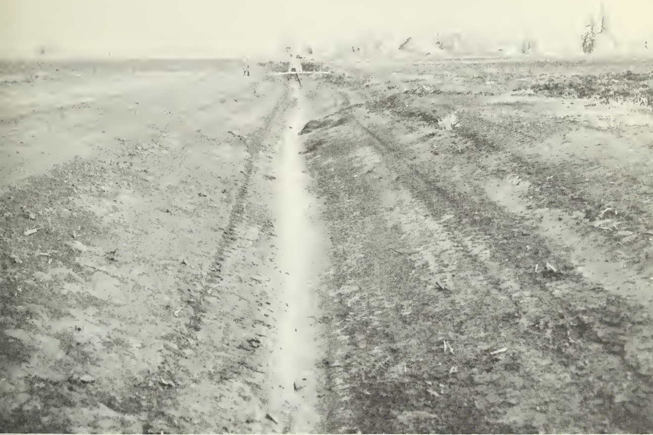
Open drain outlet for field ditches and buried tile drains. (Photo No. 0-1922-9)
