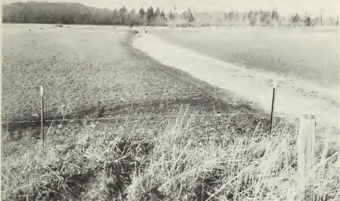
Open Channel - Waterway Outlet for Surface Drainage and subsurface drain lines. (Photo No. 0-3054-12)
