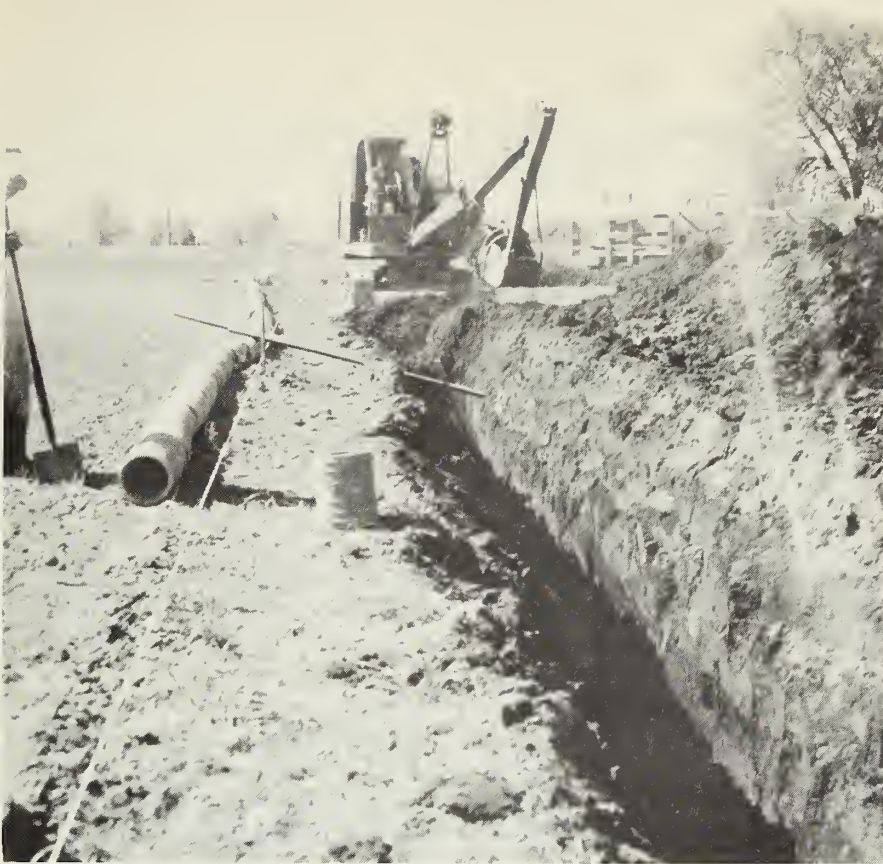
Concrete drain tile used in an inter- ceptor type drain. (Photo No. 0-522-8)
