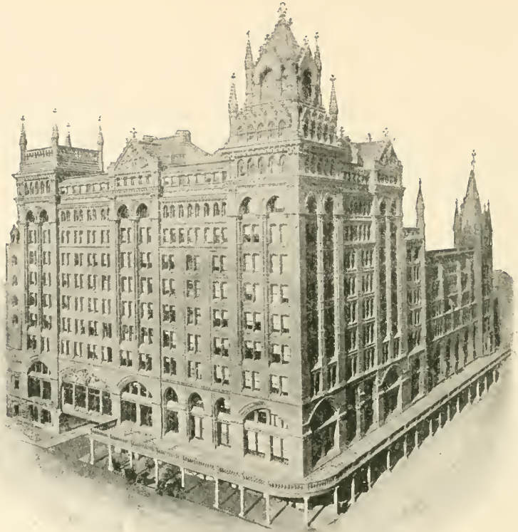
BROAD STREET STATION, PHILADELPHIA.
