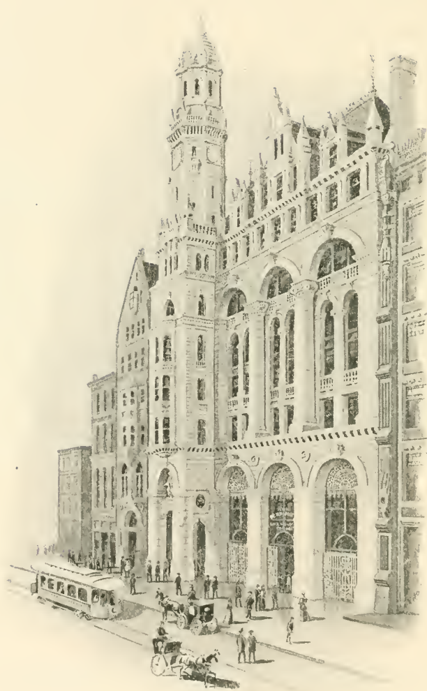
PENN MUTUAL BUILDING.
