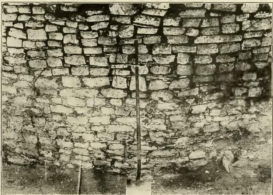
b. MASONRY IN STONE RUIN AT SITE NO. 20
