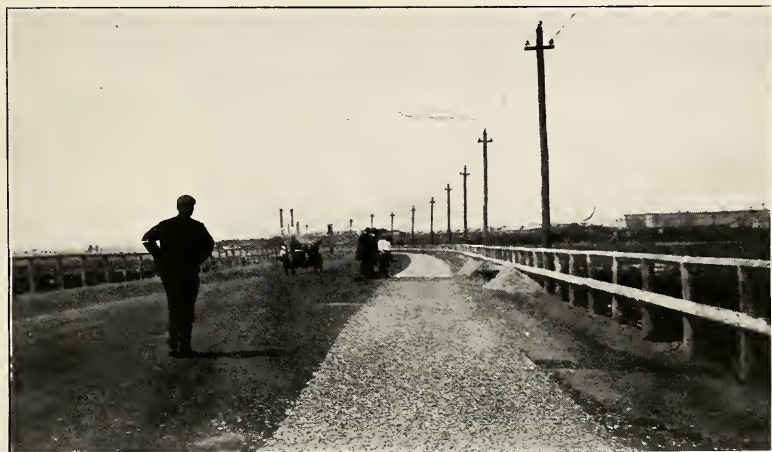
SPRAYED WITH TAR, PARTIALLY COVERED.
