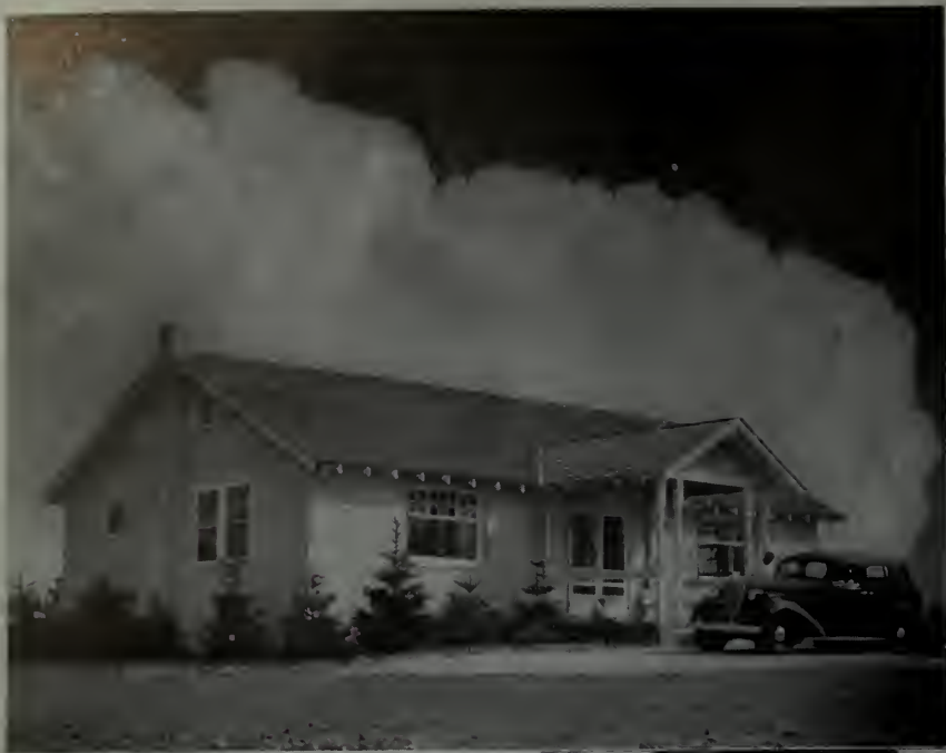
The new dairy cottage at Bonnie View Farms serves as the retail outlet for products
