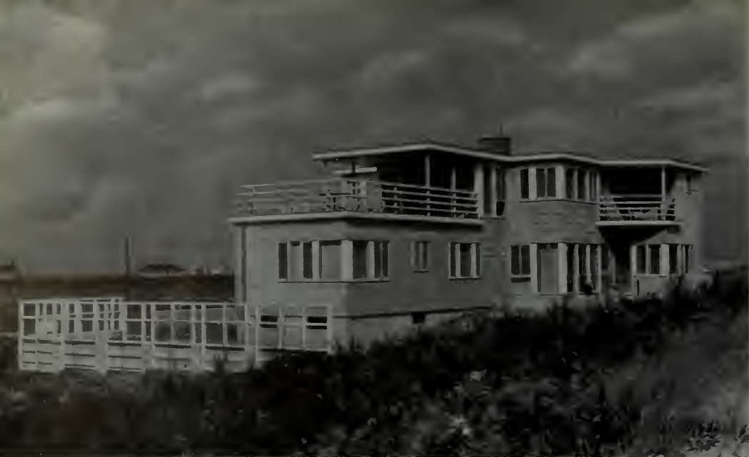
Above: The southern exposure shows the glass walls which protect the garden on the garage and basement level of the house
