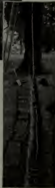
By extending the "ground" cable well beyond the root system, this part of the tree, which is just as susceptible to damage as the trunk limbs and branches, is also protected.
