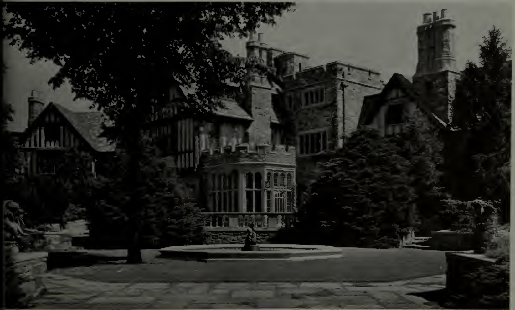
The southwestern aspect of the building centers around the breakfast room and the beautiful intimate garden—upon which it opens
