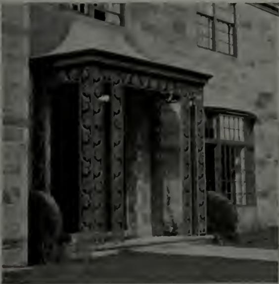
Veranda Design No. 72 as used on residence of J. Stanley Reeve, Esq., Haverford, Pa. Shepard and Stearns, Architects.
