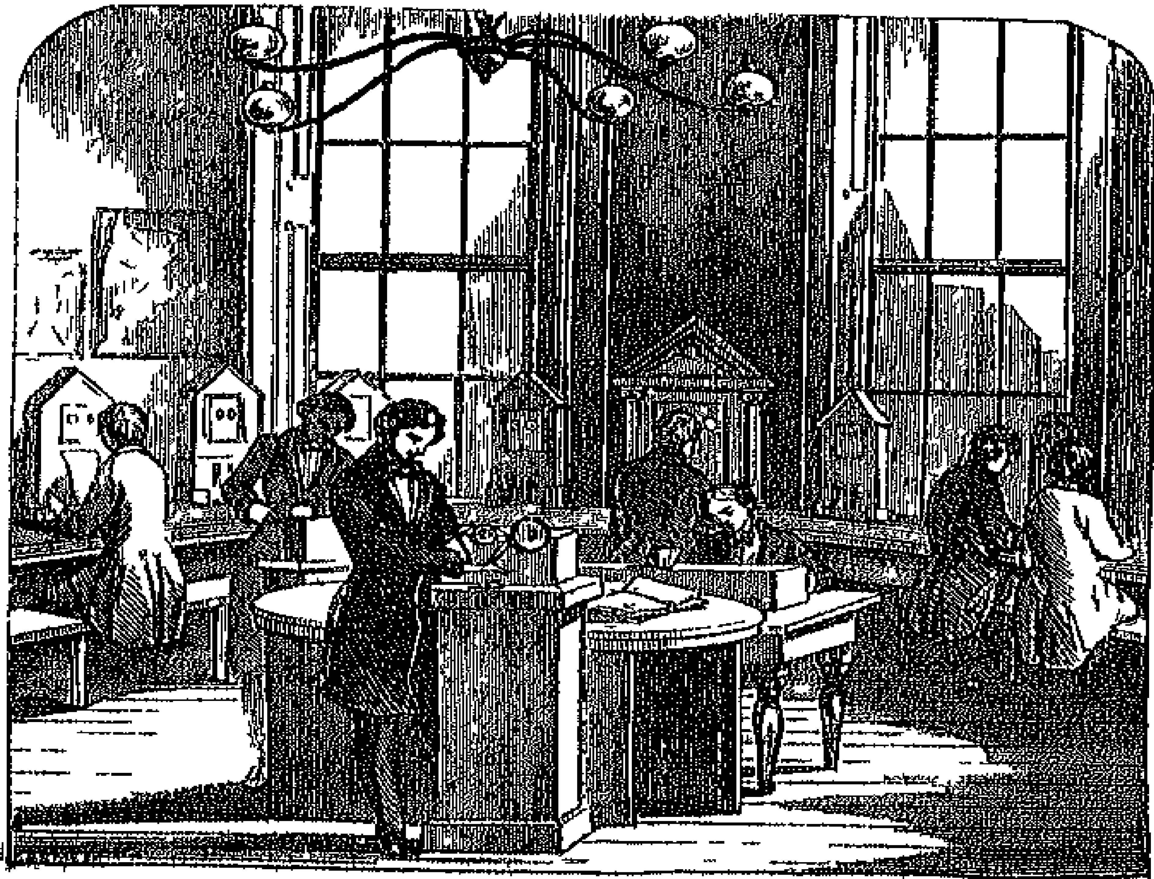
INSTRUMENT ROOM, ELECTRIC TELEGRAPH OFFICE, CHANNING CROSS
