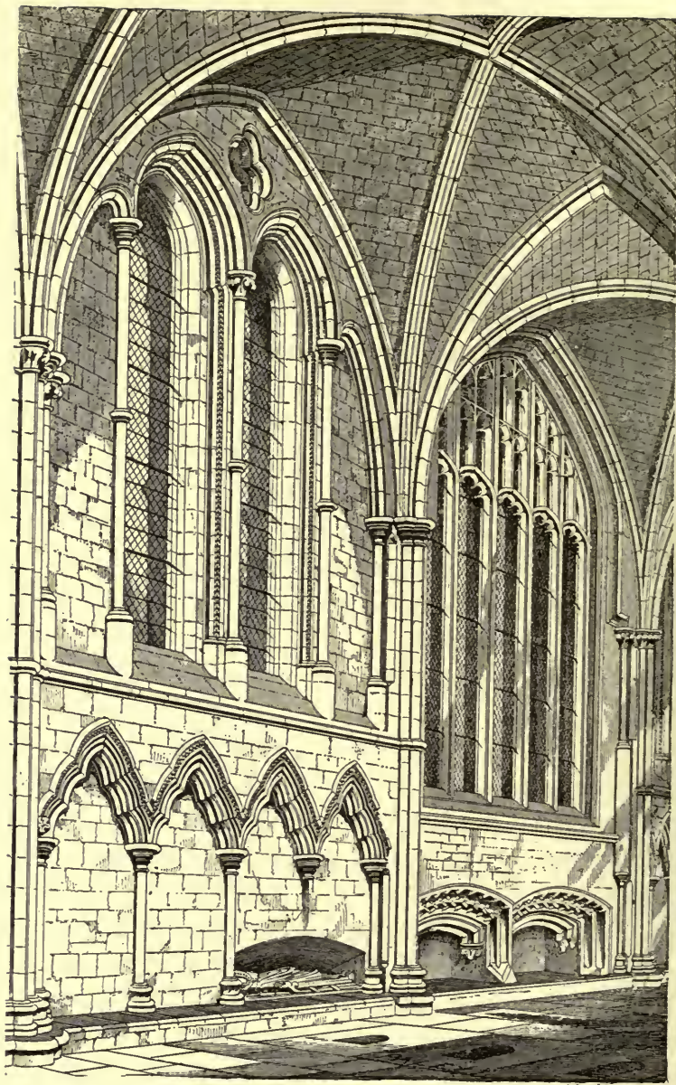
FIG. 136. Carlisle, England: Cathedral. Two bays of north aisle of choir.
