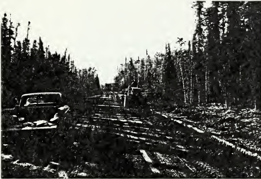
Alternate campground road built by the U.S. Army as a field exercise and bicentennial project 1977
