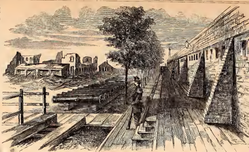
VIEW IN GOSPORT NAVY YARD, SHOWING THE WALLS OF THE LAND FINISHED FOR MASONRY, THE BEAMS OF THE WORK-SHOPS BURNED BY THE REBELS, AND THE GUNS FIXED UP FROM THE WRECKED VESSELS.
