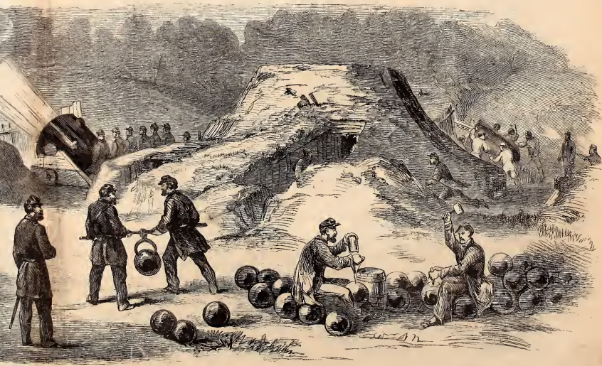
Magazine. Filling the Shell with its bursting charge. Driving the Fuse Plug. Pointing a Mortar.
