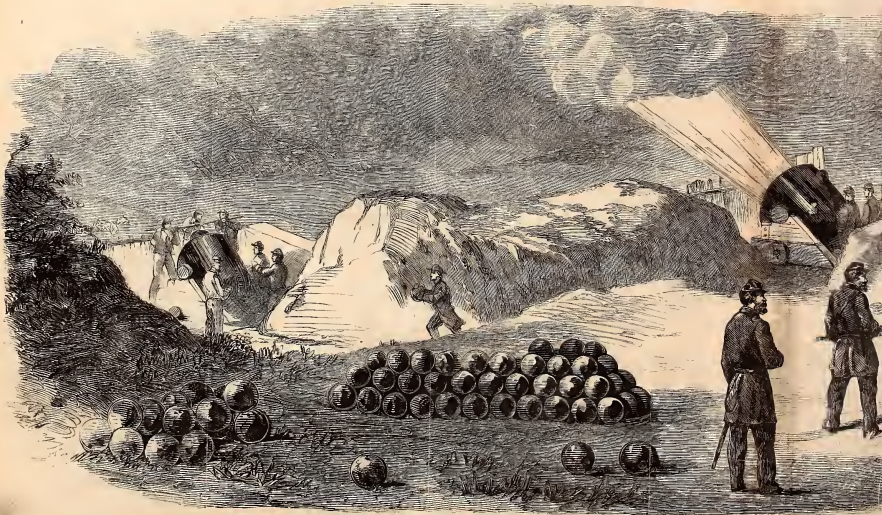
Loading a Mortar.
