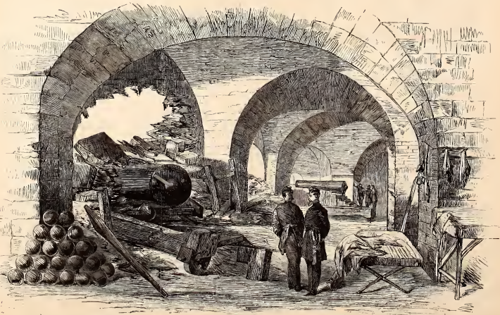
CAPTURE OF FORT PULASKI—INTERIOR VIEW OF CASEMATE, SHOWING BREACH MADE BY THE NATIONAL BATTERERS.—FROM A SKETCH BY OUR SPECIAL ARTIST, W. T. CRANE.—SEE PAGE 46.
