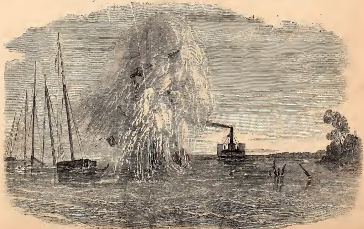
THE WAR IN NORTH CAROLINA.—REMOVING BURNED SCISSORS FROM ONE OF THE BARRIERS TO OBTAIN THE DAMAGE OF THE FEDERAL GOVERNMENT, UNDER THE SUPERINTENDENCE OF CAPT. HAYDEN, OF THE NEW YORK GUERRILLAS ENGINEERING COMPANY.—FROM A SKETCH BY OUR SPECIAL ARTIST, MR. J. H. SCHILL.—SEE PAGE 215.
