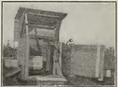
Frame work of scale house.
