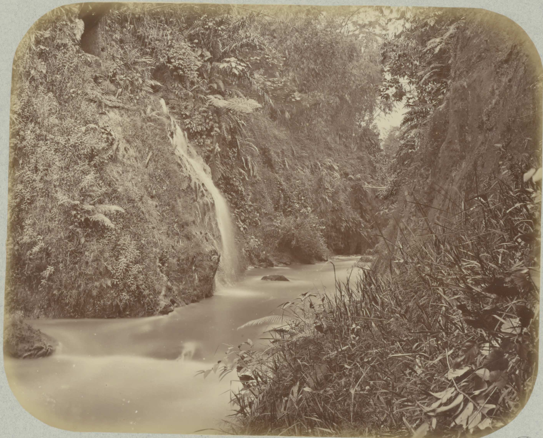
View from the bridge near the Railway station Britenzorg
