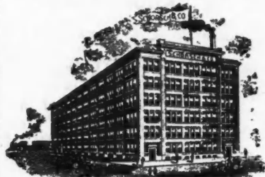
FACTORY 132 ND TO 133 RD ST. & BROOK AVE
