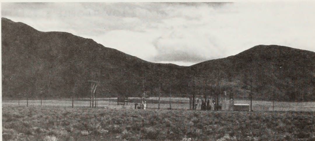
Existing 120 kv substation, Oreana, Nevada.
