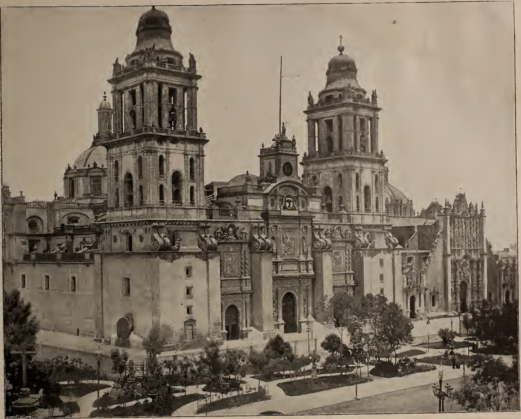
CATHEDRAL AT CITY OF MEXICO.—This great Cathedral is in the form of a Latin cross, and over the central arches rises a magnificent dome, decorated by the most celebrated artists. The dimensions of the church are length, three hundred and fifty-four feet, width, one hundred and seventy-seven feet, height, one hundred and seventy-nine feet. There are five naves, six altars, and fourteen chapels. The massive railing about the entrance to the choir is a curiosity in metal as well as art. It is made of a composition of gold, silver and copper and came from Chiua. Along the passage from the choir to the altar are sixty or seventy small figures made of the same brilliant metal, which serve as light bearers. The pulpits and the huge holy-water basins are of onyx. Of the fourteen chapels, seven are on each side. In one of these is the tomb of Iturbide. Of the six altars the most beautiful is the altar of the Kings. Below this rest the remains of some of the viceroys and of the four patriots, Hidalgo, Aldama, Allende and Jimenez who were executed in Chihuahua. The Cathedral stands on the site of the Aztec temple, which was destroyed by Cortez. It was begun in 1573 and finished in 1667. The towers were finished in 1791, at a cost of $300,000.
