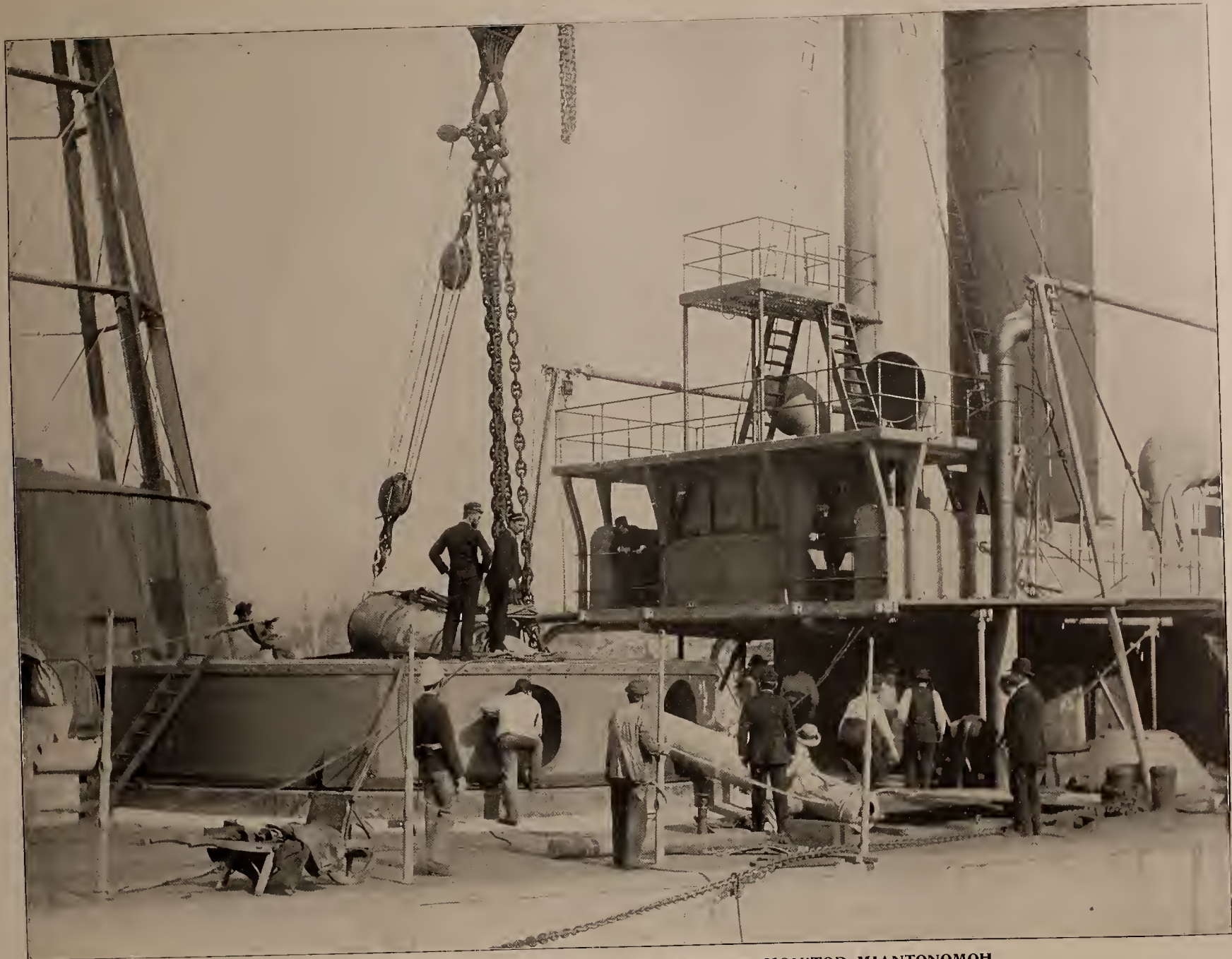
PLACING A TEN-INCH GUN IN A TURRET ON THE U. S. MONITOR MIANTONOMOH.
