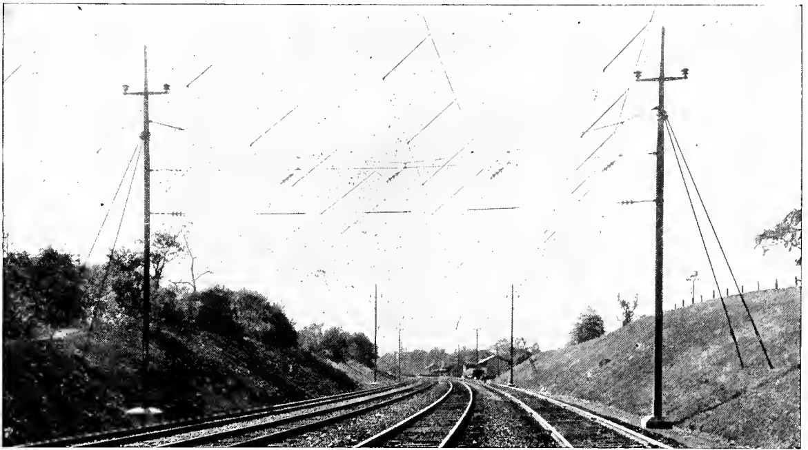
A Section of the Line Construction of the Philadelphia-Paoli Electrification on the Pennsylvania Railroad
