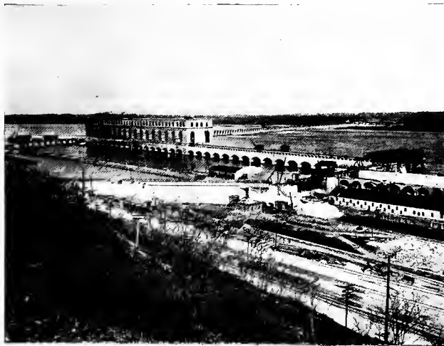
General View of Power House of the Mississippi River Power Company of Keokuk, Iowa, taken from the Iowa Side
