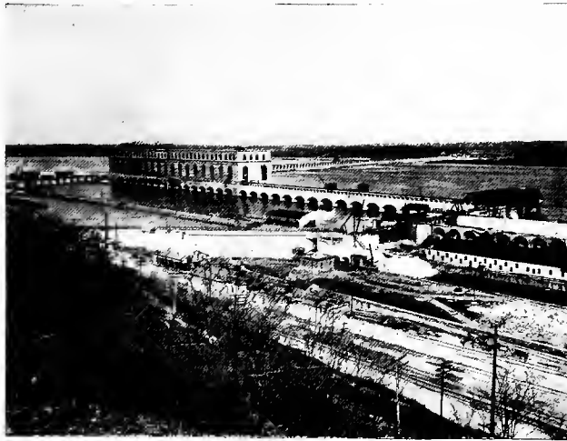
General View of Power House of the Mississippi River Power Company of Keokuk, Iowa, taken from the Iowa Side
