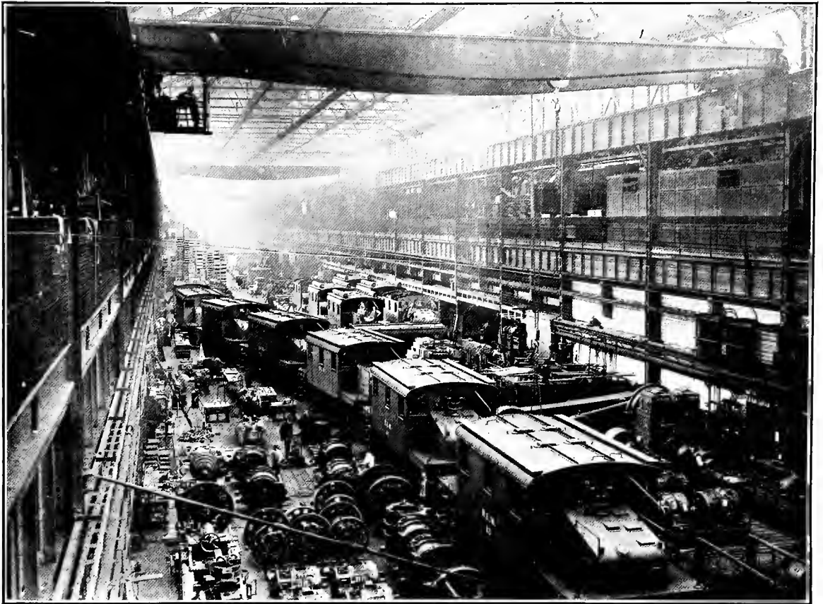
Equipping Electric Locomotives in the Westinghouse Works
