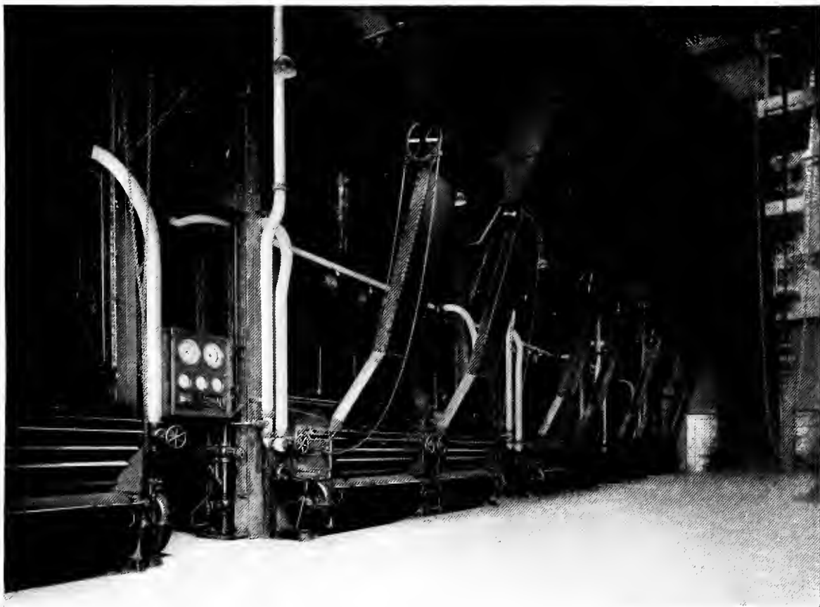
Figure 2. A Section of the Modern Boiler Room in One of the Commonwealth Edison Company's Chicago Plants as Compared with the old Pearl Street Station Shown on a Preceding Page
