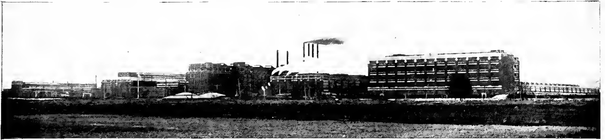
General View of the Erie, Pa., Works of the General Electric Company
