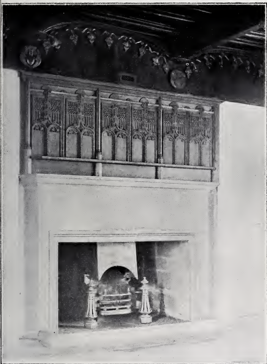
PLATE IV.—FIREPLACE IN THE PRIOR'S ROOM : THE DEANERY, CARLISLE.
